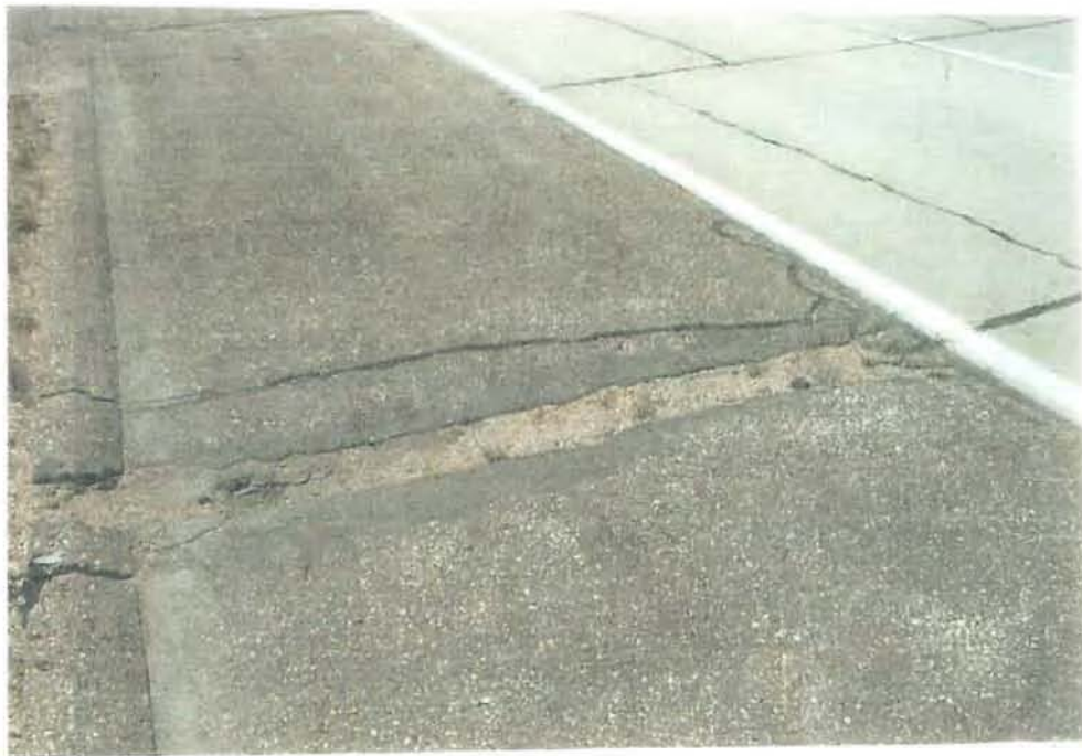
Figure 2. Pre-construction Roadway and Shoulder Condition
