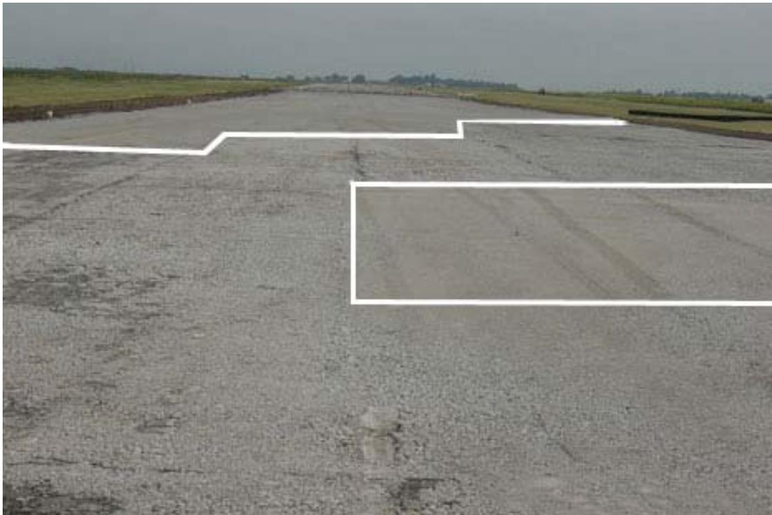
**Figure 2.10, Finished Patched Areas Outlined in White at Pratt using Crusher Run**
