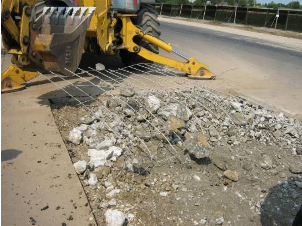
**Figure 5.2, Test Pit with Rebar Mat Substantially Debonded**
