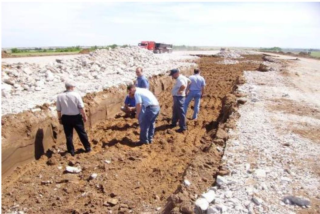
**Figure 2.12, Full-depth Excavation Deep Into Subgrade of Patched Area at Kegelman**
