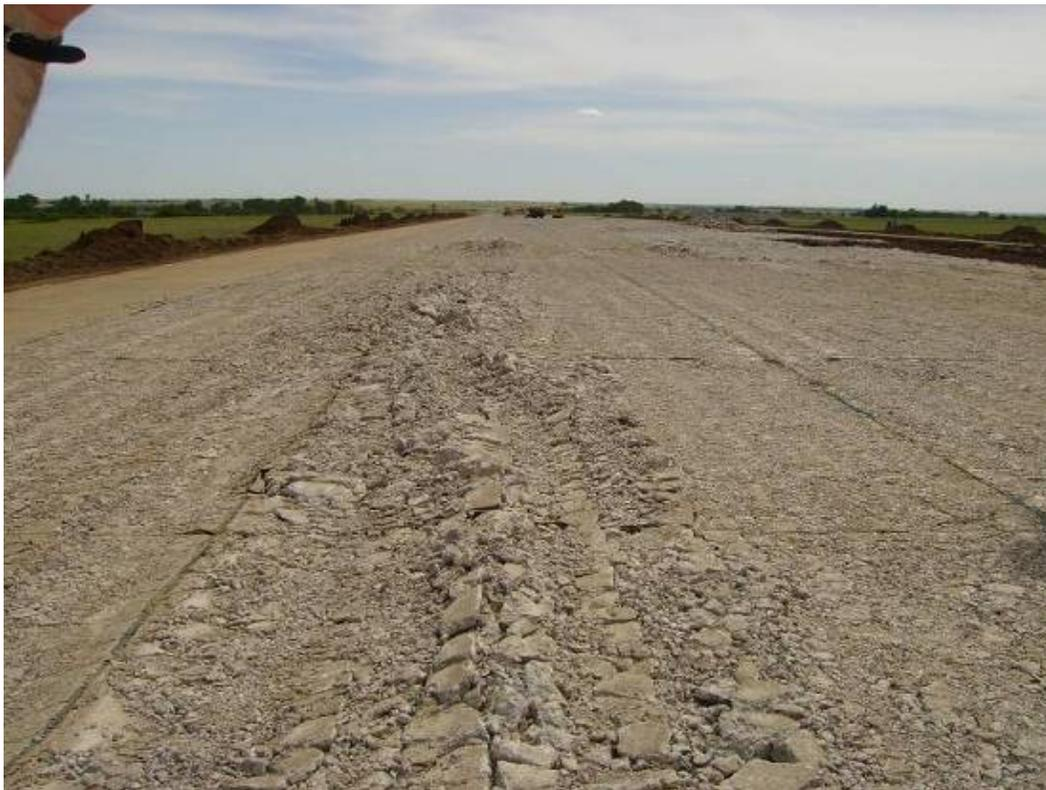
**Figure 2.11, Rutting from RPB of Unstable Area at Kegelman that Requires Excavation**
