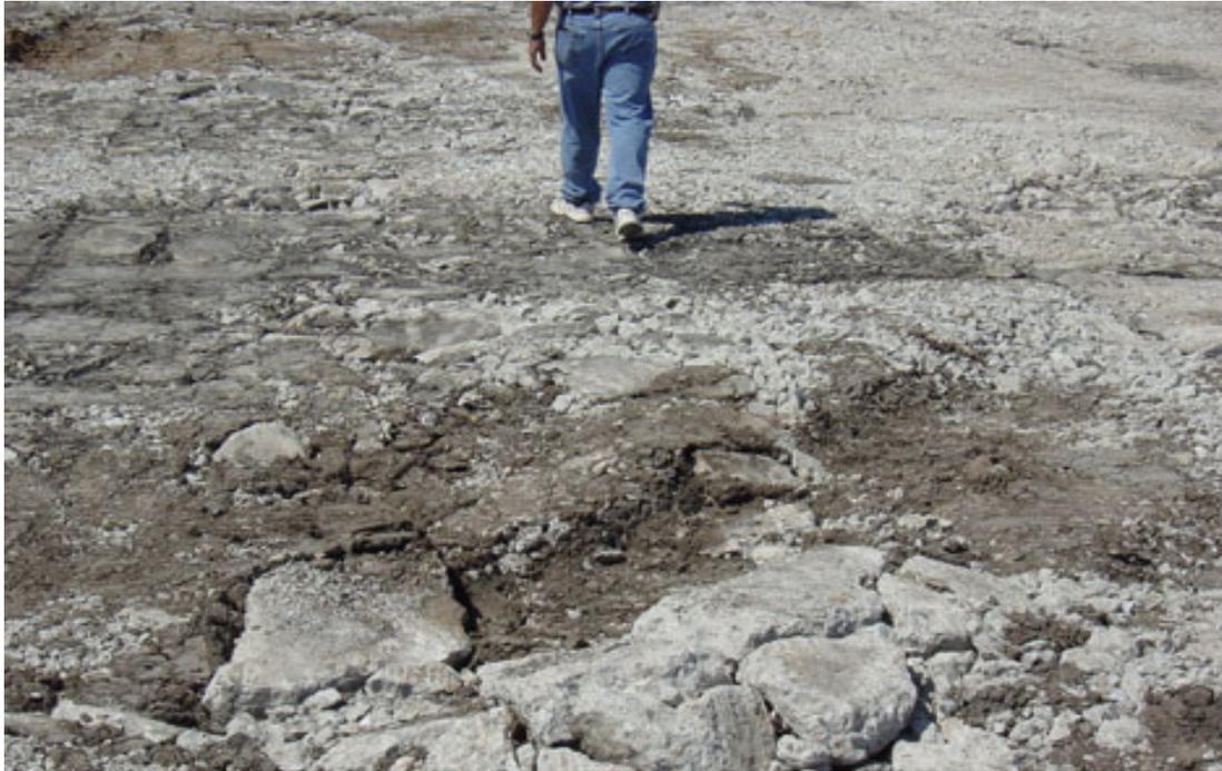
**Figure 2.7, Ineffective Rubblization (Large PCC Pieces) at Pratt Due to Weak Support**
