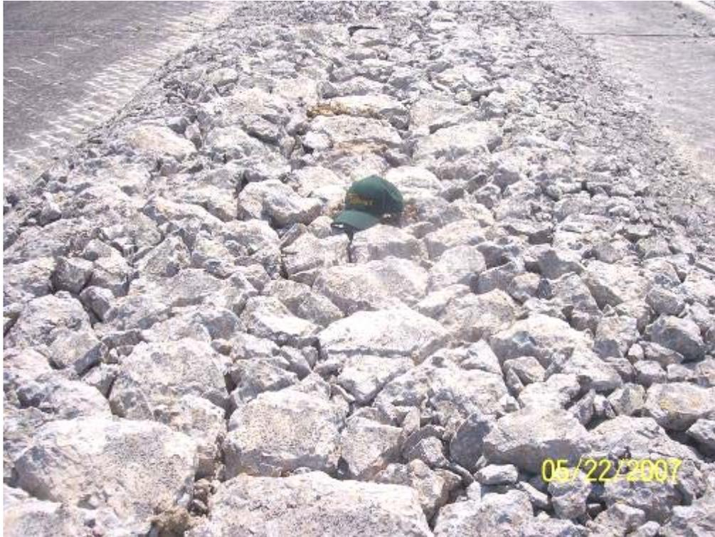
**Figure 3.9, Unacceptable Rubblization from Start-up of MHB at Tullahoma**
