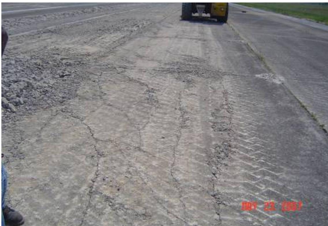
**Figure 2.13, Fractured PCC by MHB with Low Drop Ht. and Wide Spacing at Tullahoma**
