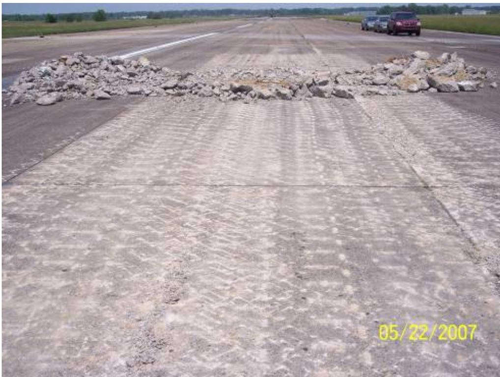
**Figure 3.10, Result of “Modified Rubblization” Process after Z-grid at Tullahoma**
