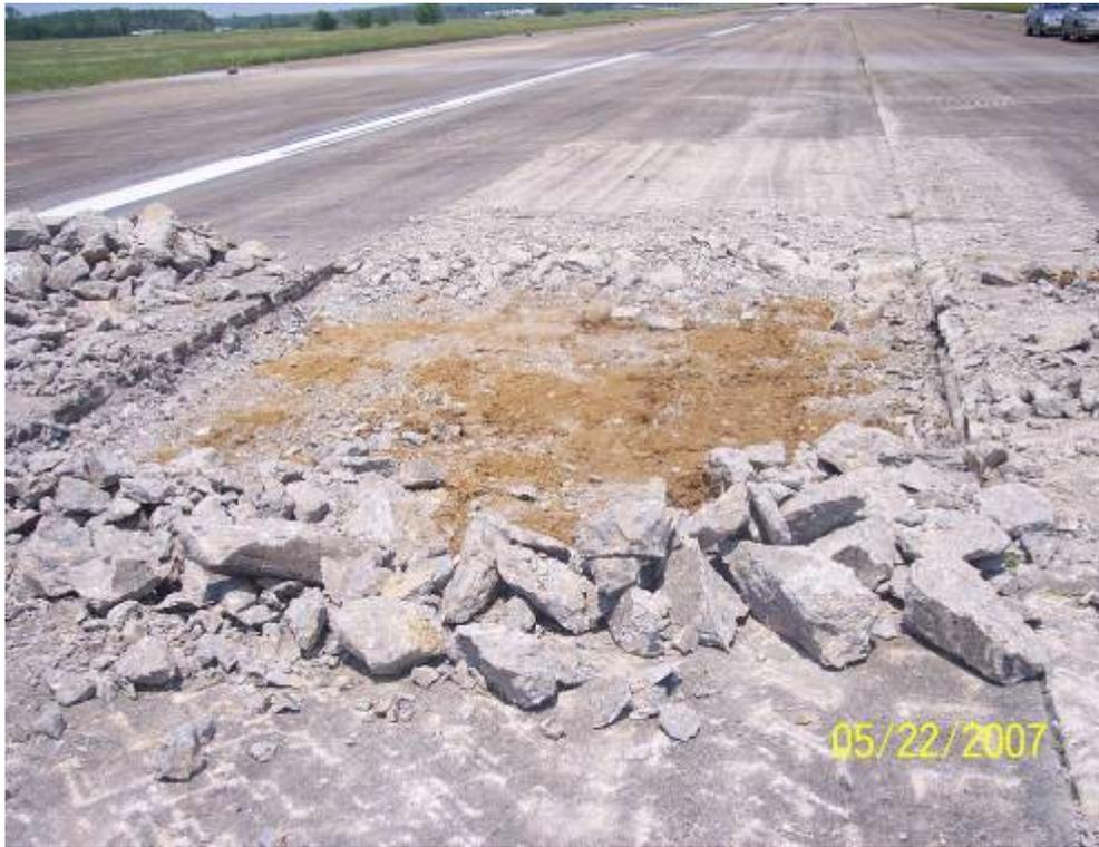
**Figure 3.11, Test Pits from “Modified Rubblization” at Tullahoma**
