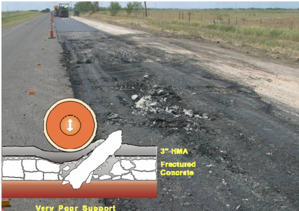
**Figure 3.7, Shifting of Rubblized PCC from Paving Operations on Texas SH 70**
