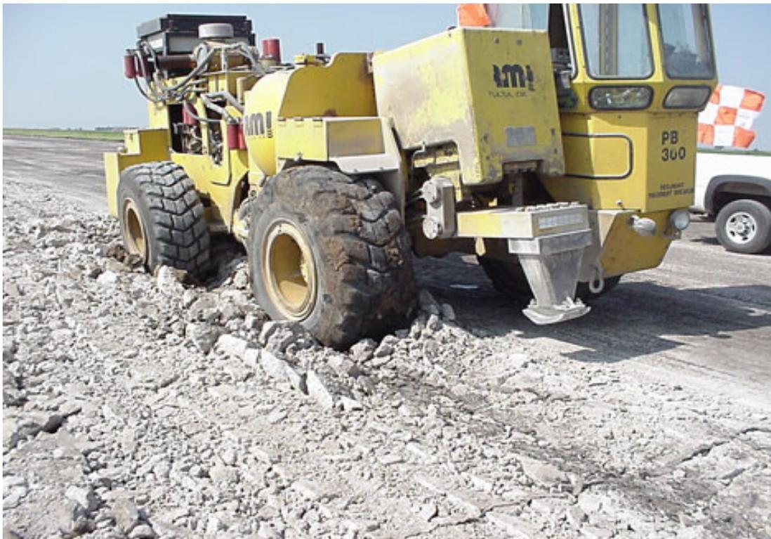
**Figure 2.8, RPB with High Flotation Tires Stuck in Unstable Area at Pratt**
