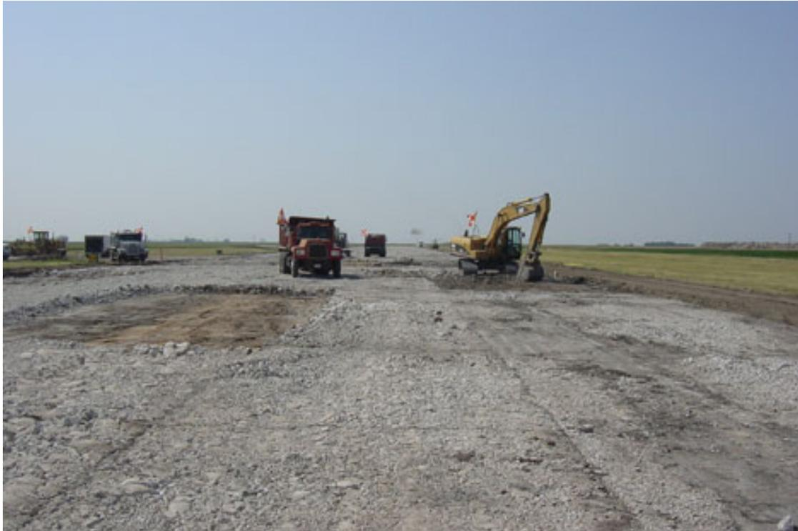
**Figure 2.9, Excavation of Ineffective Rubblized Areas at Pratt for Full-depth Patch**
