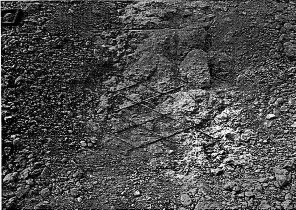
**Figure 2.2, Photo Showing Partial Debonding of Temperature Steel [Baladi et al, 2002]**
