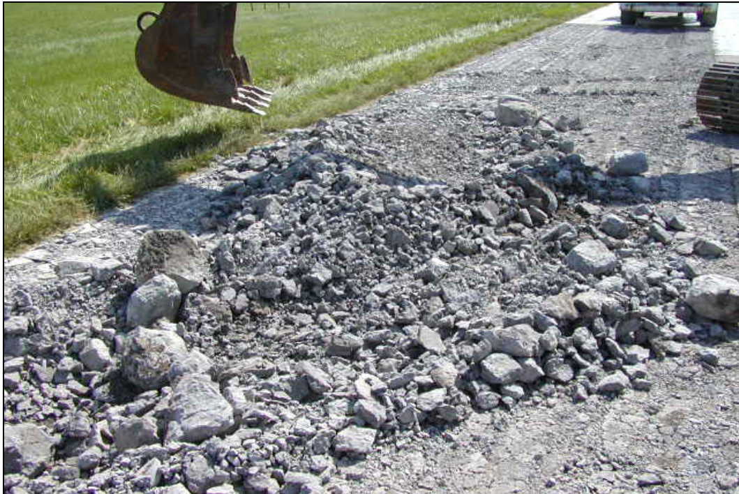
Figure 5. Inspection Test Pit
