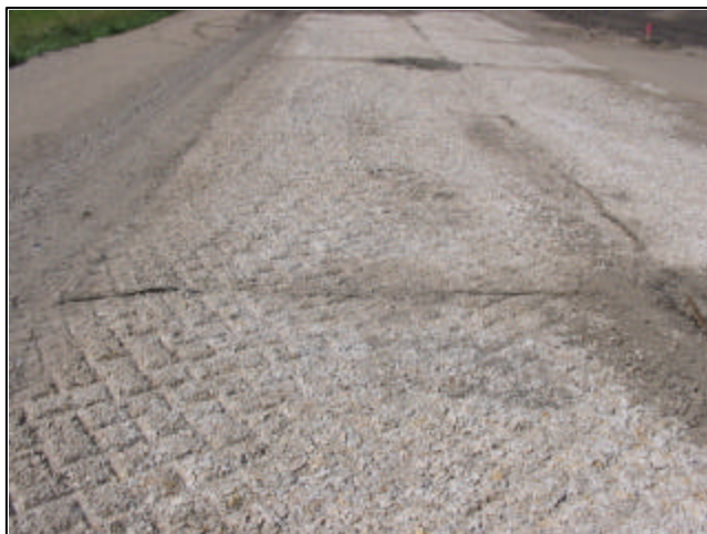
Rubblizing the deteriorated pcc on CSAH 16 prior to HMA overlay.
