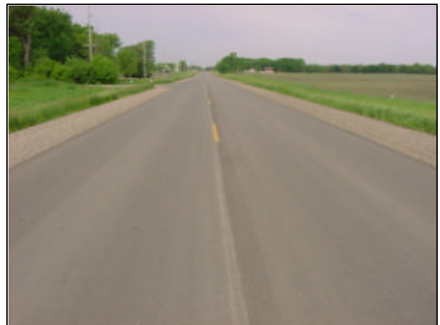
CSAH 16 prior to final 1½-inch wear course.
