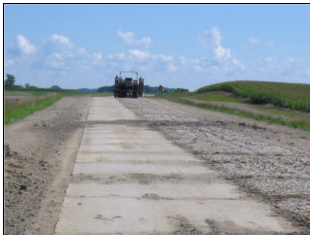
Rubblizing the deteriorated pcc on CSAH 16 prior to HMA overlay.
