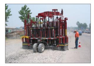
Developed by an affiliate of Wisconsin's Antigo Construction Company, this multiple drop hammer machine reduces concrete pavement to rubble in minutes. The aggregate-like rubble is left in place and a PCC overlay is placed over it. Photo courtesy of Antigo Construction.
