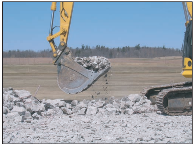
Excavator removing broken jointed reinforced concrete
