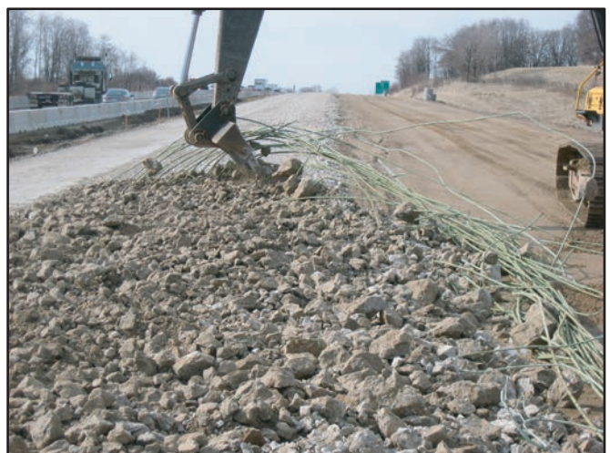
Excavator raking rebar out of the broken concrete
