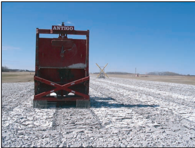
8600 breaking airport runway for removal
