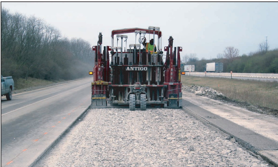
MHB Badger Breaker® rubblizing a motorway
