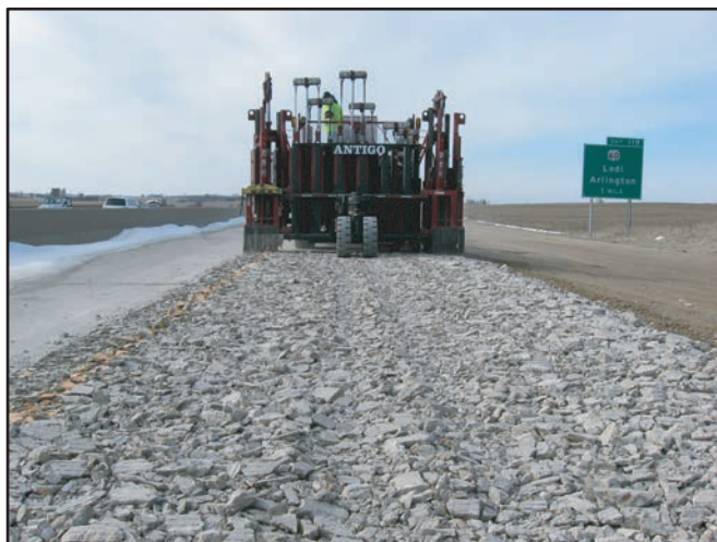
MHB breaking continuously reinforced concrete to allow for rebar removal
