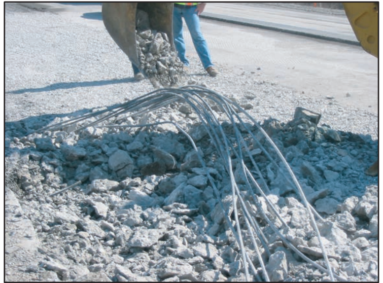
Continuously reinforced concrete pavement
