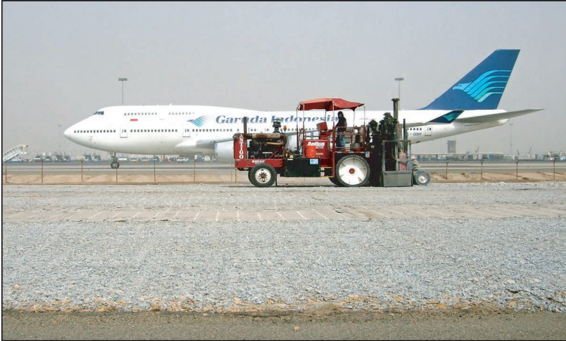
MHB Badger Breaker® rubblizing an airport runway
