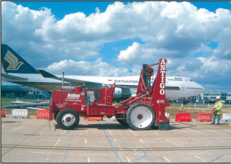
Typical airport cracking operation using an 8600 Badger Breaker®
