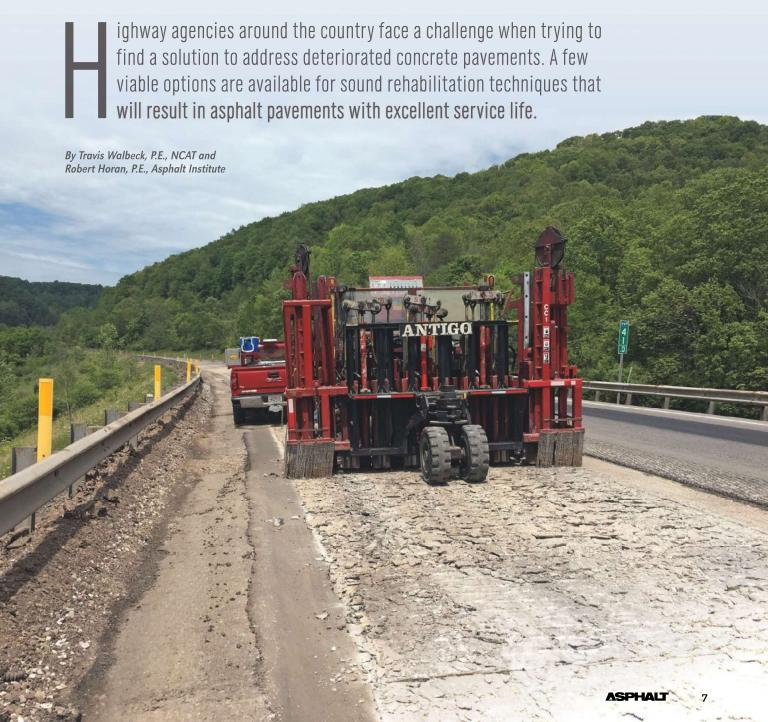
Removing the old concrete and replacing it with new portland cement concrete (PCC) pavement is an expensive option. Removing the concrete and constructing a new hot mix asphalt (HMA) pavement is normally less expensive, but it still incurs the cost of removing and wasting the old pavement. Overlaying the existing concrete with HMA is relatively inexpensive. However, with this option, reflective cracking can be a maintenance problem.
