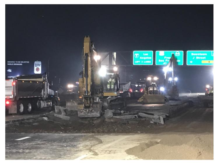
Crack-and-seat overlays can only be used on concrete panels in somewhat decent shape, Mihal said. For panels that had failed, the Granite crew had to remove and replace them before cracking the new panels alongside the old ones.
