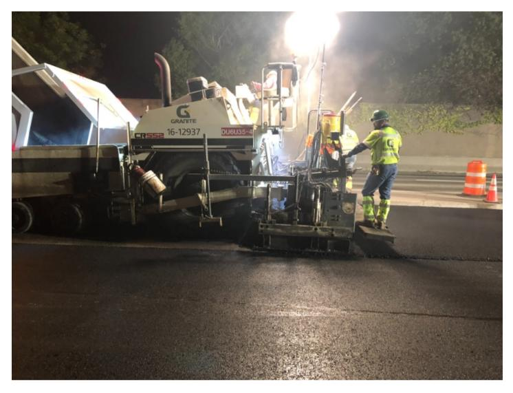
Most of the paving on the I-5 job was performed with Granite's Cat AP1055F track paver and Cedar Rapids 522 track paver, with a variety of Sakai, Hamm, and Cat rollers.
