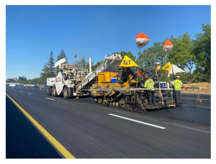
On top of the cracked and seated concrete, Granite's crew placed a 1.2-inch leveling course followed by a geosynthetic pavement interlayer (GPI), 5.4 inches of intermediate mix, 2.4 inches of a high-polymer surface course mix and 1.2 inches of rubberized OGFC.
