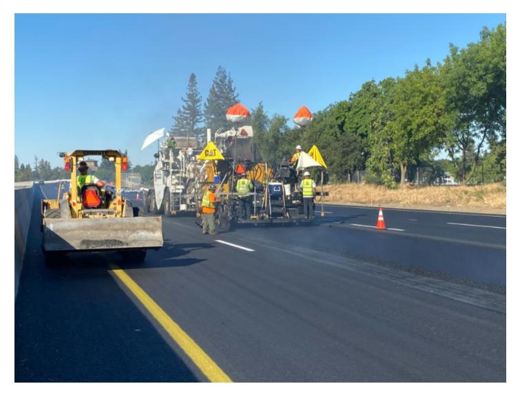
As the crews paved the overlay, they tapered it over the full-depth asphalt pavement section as they approached the transition sections. "When all was said and done, we didn't throw away nearly as much material and were also able to utilize a more efficient construction method using perpetual asphalt pavement as opposed to precast concrete," Curtis said.
