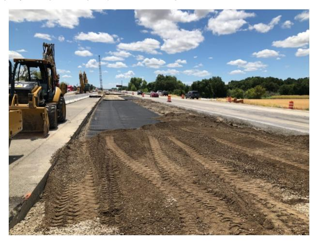
Although Curtis said there are differences throughout the pavement design for the widening sections, the standard outside layer on main sections included a Triax geogrid layer in contact with the subgrade, 1 foot of Class 2 aggregate base, 2.4 inches of a rich bottom mix, 8.4 inches of intermediate course, a 2.4-inch surface course, then 1.2 inches of OGFC.
