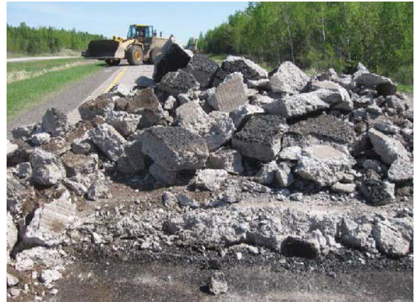
Removing upper layer of concrete
