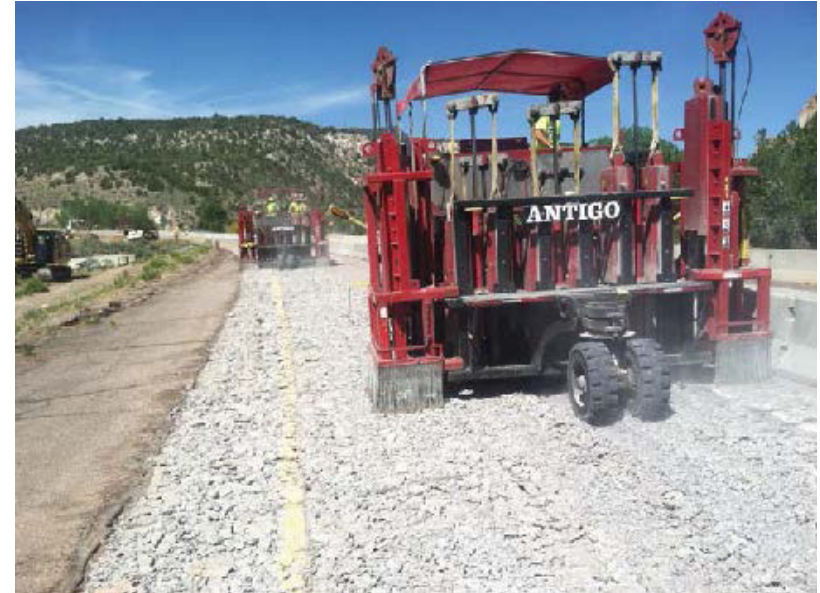
MHB Badger Breaker® rubblizing concrete
