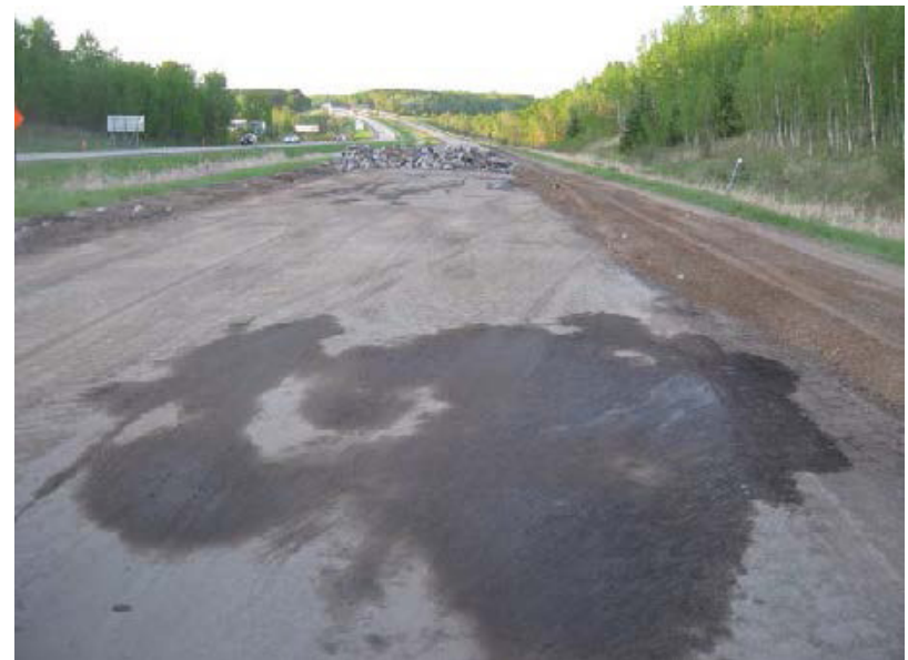
Underlying concrete layer not damaged after breaking and removing upper layers of concrete and asphalt
