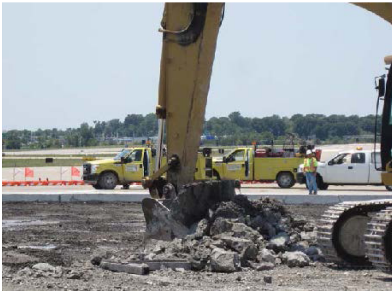
Removing upper layer of concrete and asphalt layer
