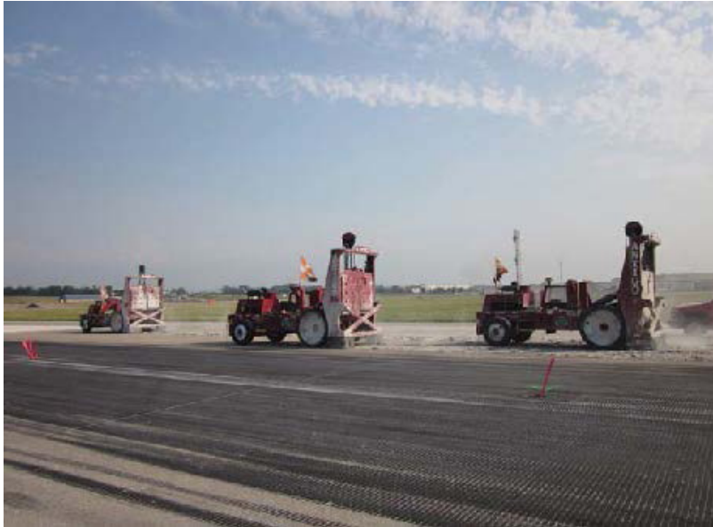
8600 Badger Breakers® breaking upper layer of concrete
