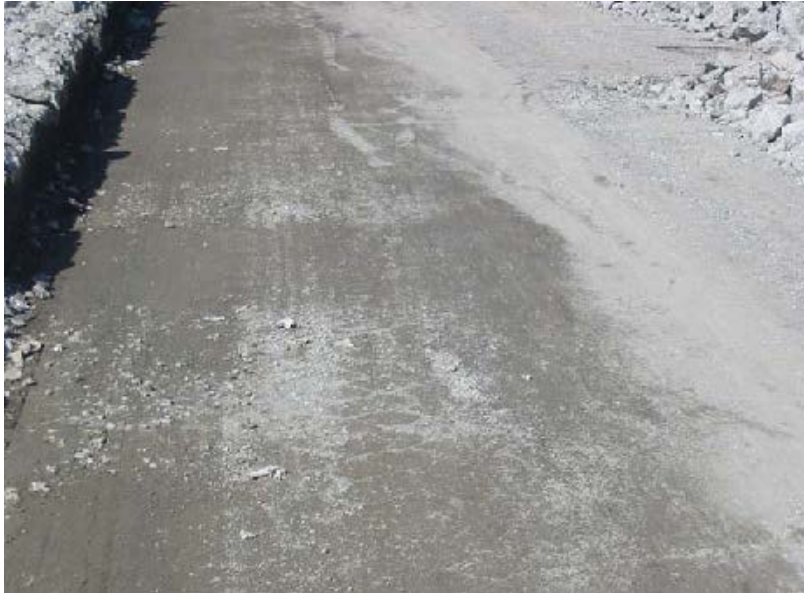
Lower layers not damaged after breaking and removing upper layer
