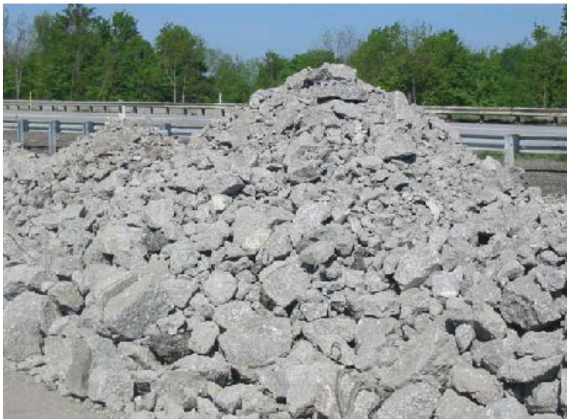
Concrete removed and windrowed
