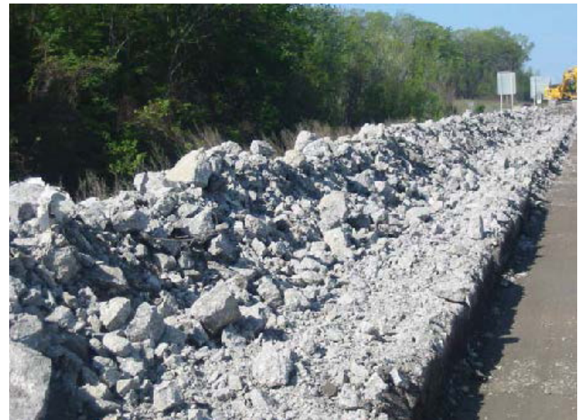
Concrete removed and windrowed
