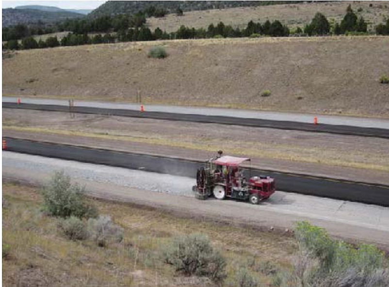
MHB Badger Breaker® rubblizing concrete
