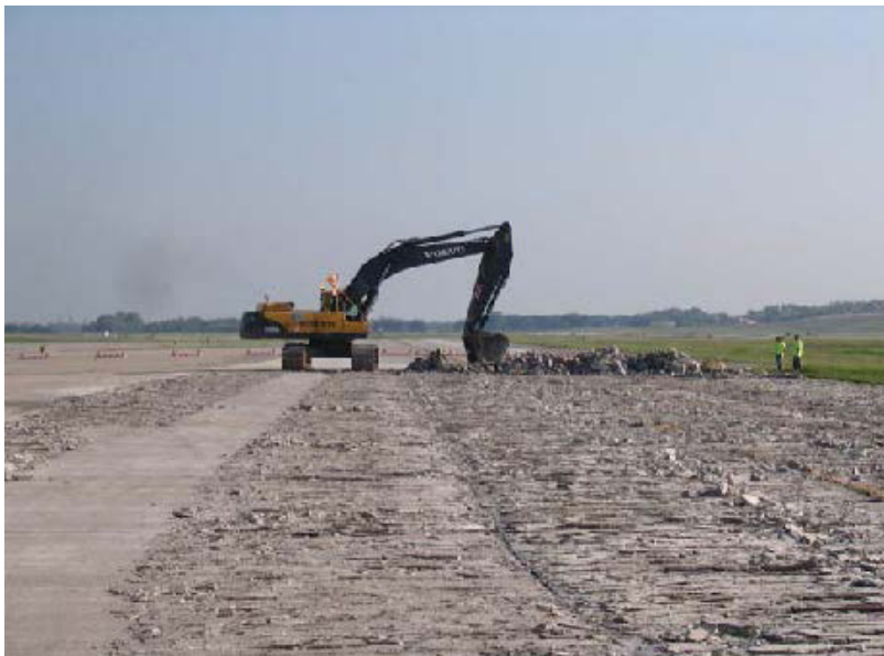
Removing concrete
