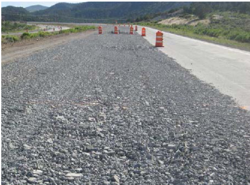
Surface of rubblized concrete layer
