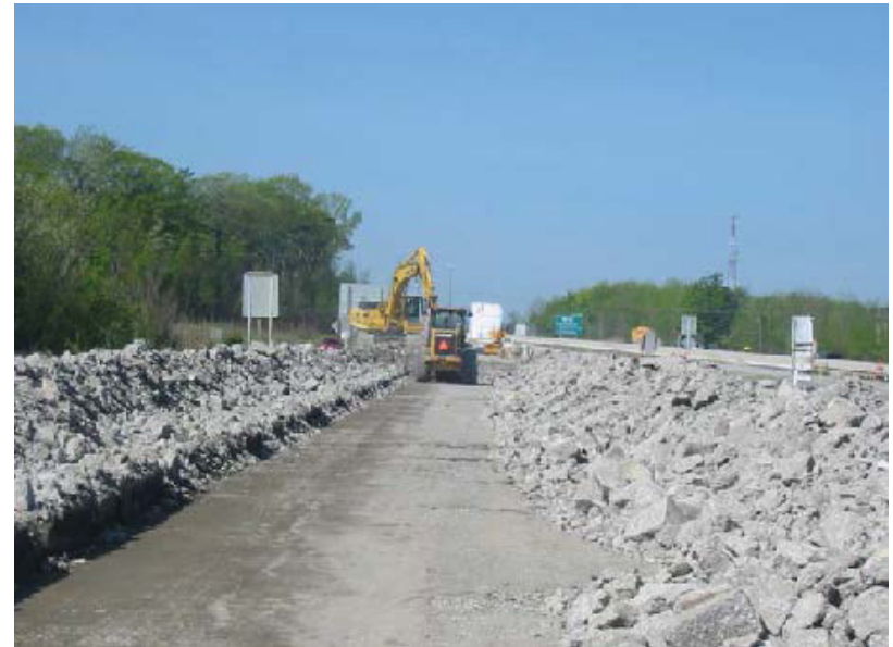
Removing upper layer of concrete
