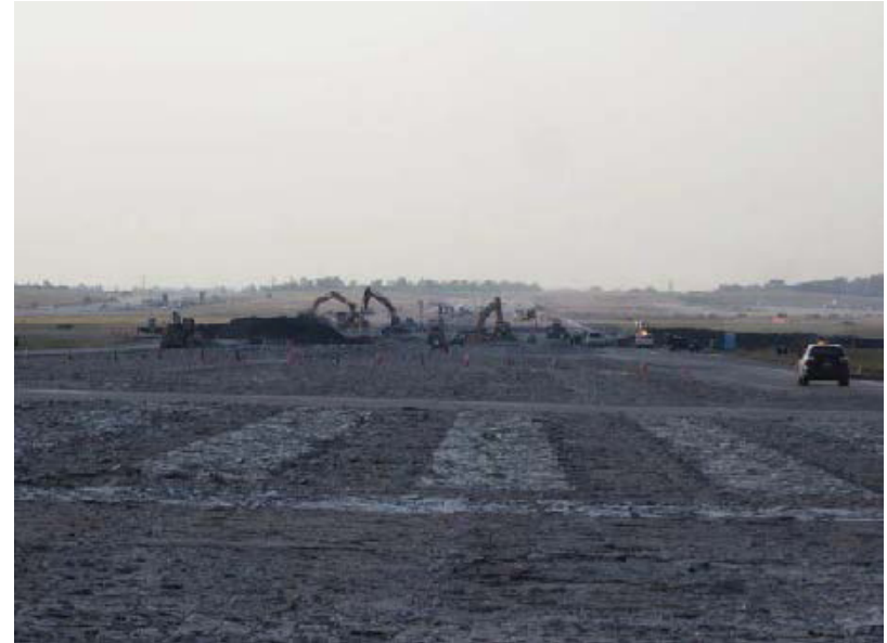
Upper layer of broken concrete
