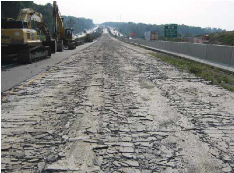
Upper layer of concrete broken with T8600 Badger Breaker®
