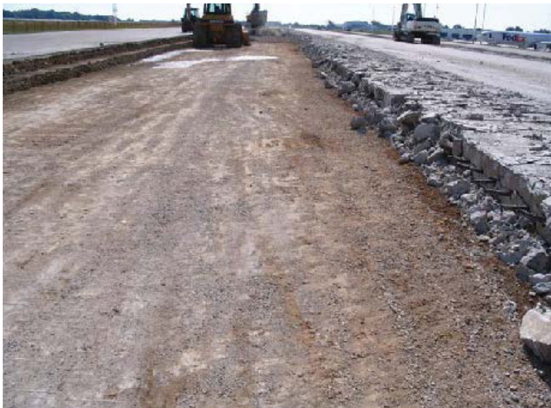
Underlying CTB layer not damaged (required 2nd pass to break CTB layer for removal)
