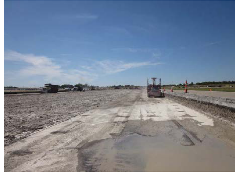
Breaking lower layer of concrete
