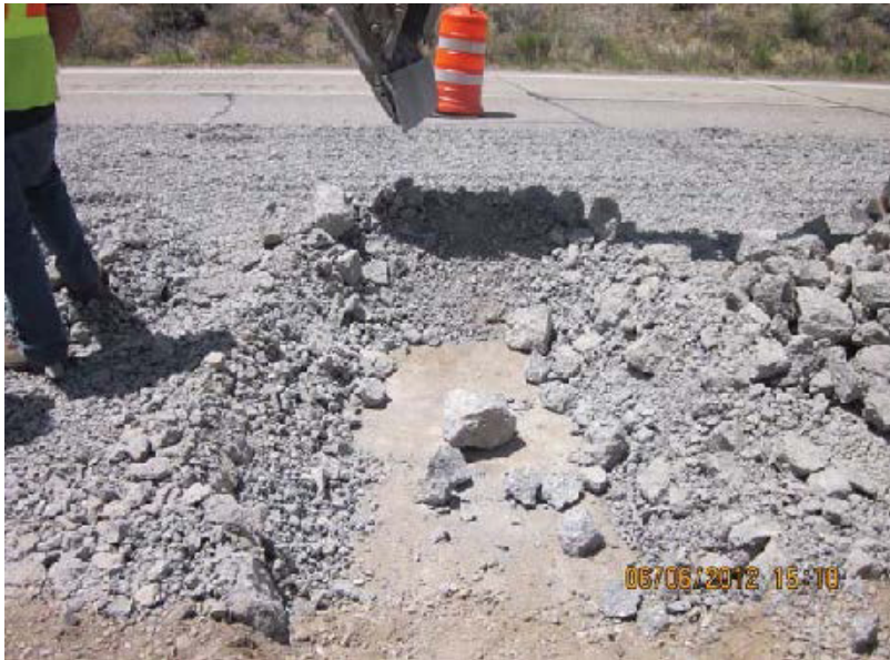
Underlying lean concrete base not damaged after rubblizing concrete
