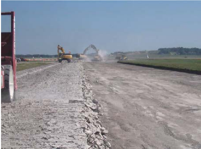
Underlying asphalt layer on right not damaged after breaking and removing upper layer
