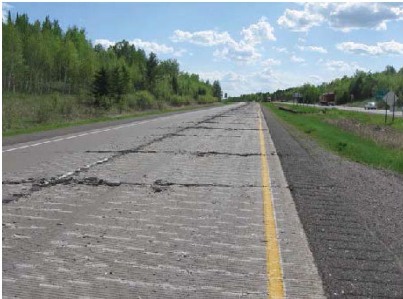
MHB Badger Breaker® breaking pattern
