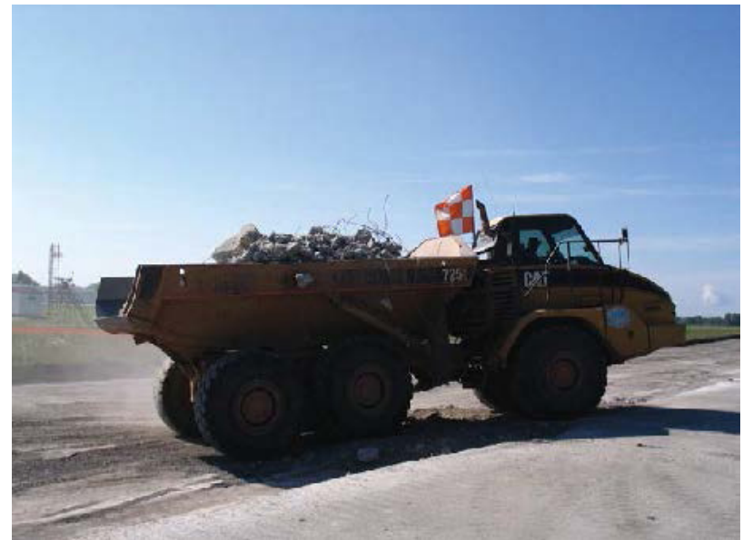
Hauling broken concrete
