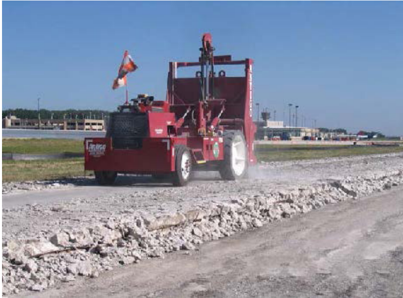
8600 Badger Breaker® breaking concrete
