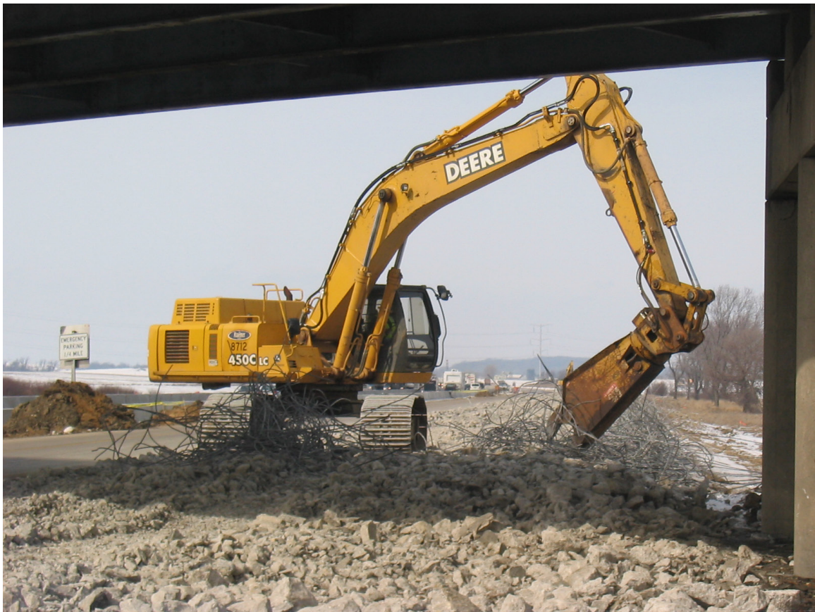
Excavator with shears attachment cutting reinforcing bar to manageable size for hauling to recycling center.
