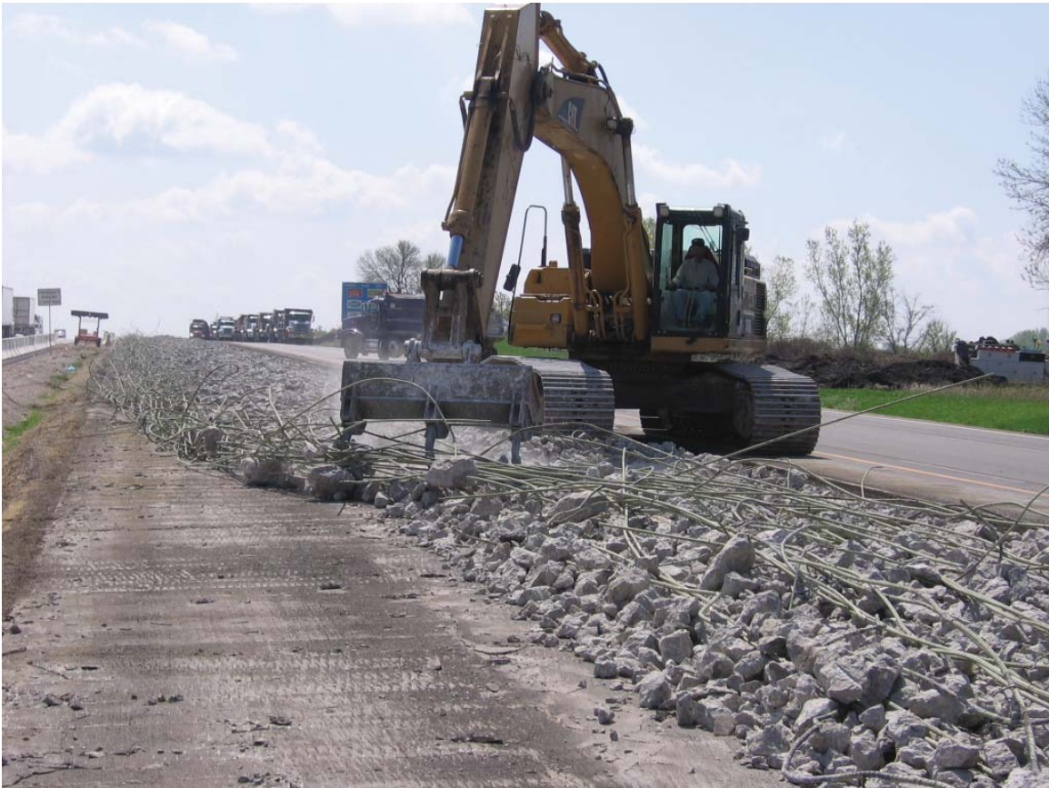
Excavator with rake attachment raking reinforcing bar from the broken concrete.
