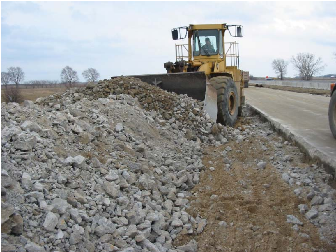
Front end loader picking up broken concrete.
