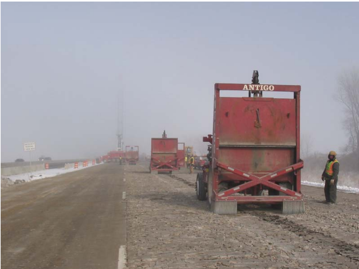
Hammers striking concrete at approximately 6-inch intervals.
