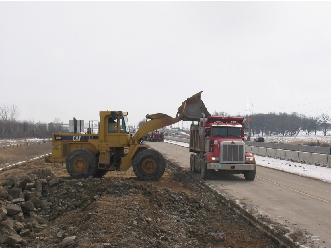
Front end loader loading broken concrete in dump truck for transport to crushing site.
