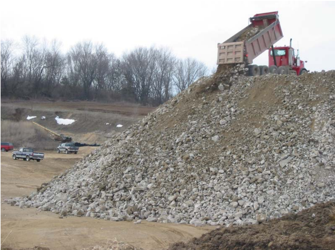
Stockpile of broken concrete at crushing site.
