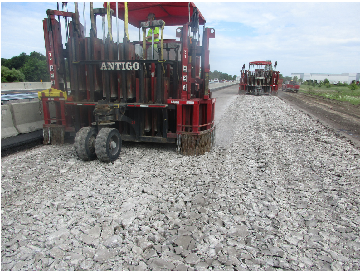
Two MHB Badger Breakers® breaking continuously reinforced concrete pavement.
