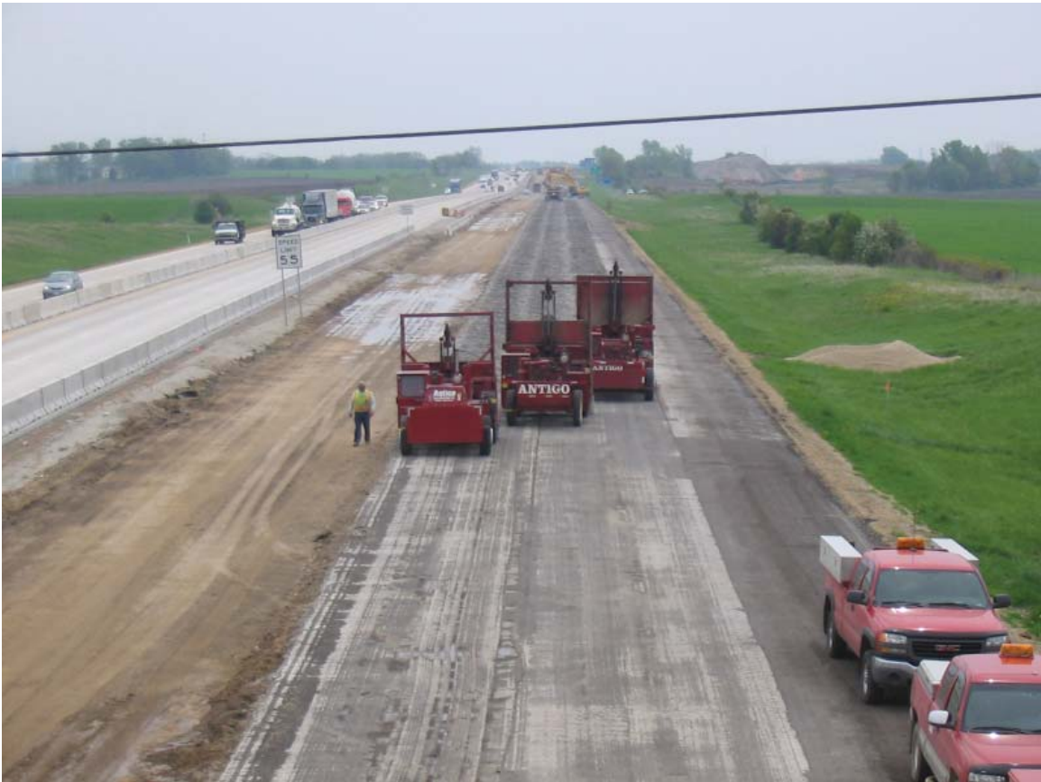
Three 8600 Badger Breakers® breaking continuously reinforced concrete pavement.
