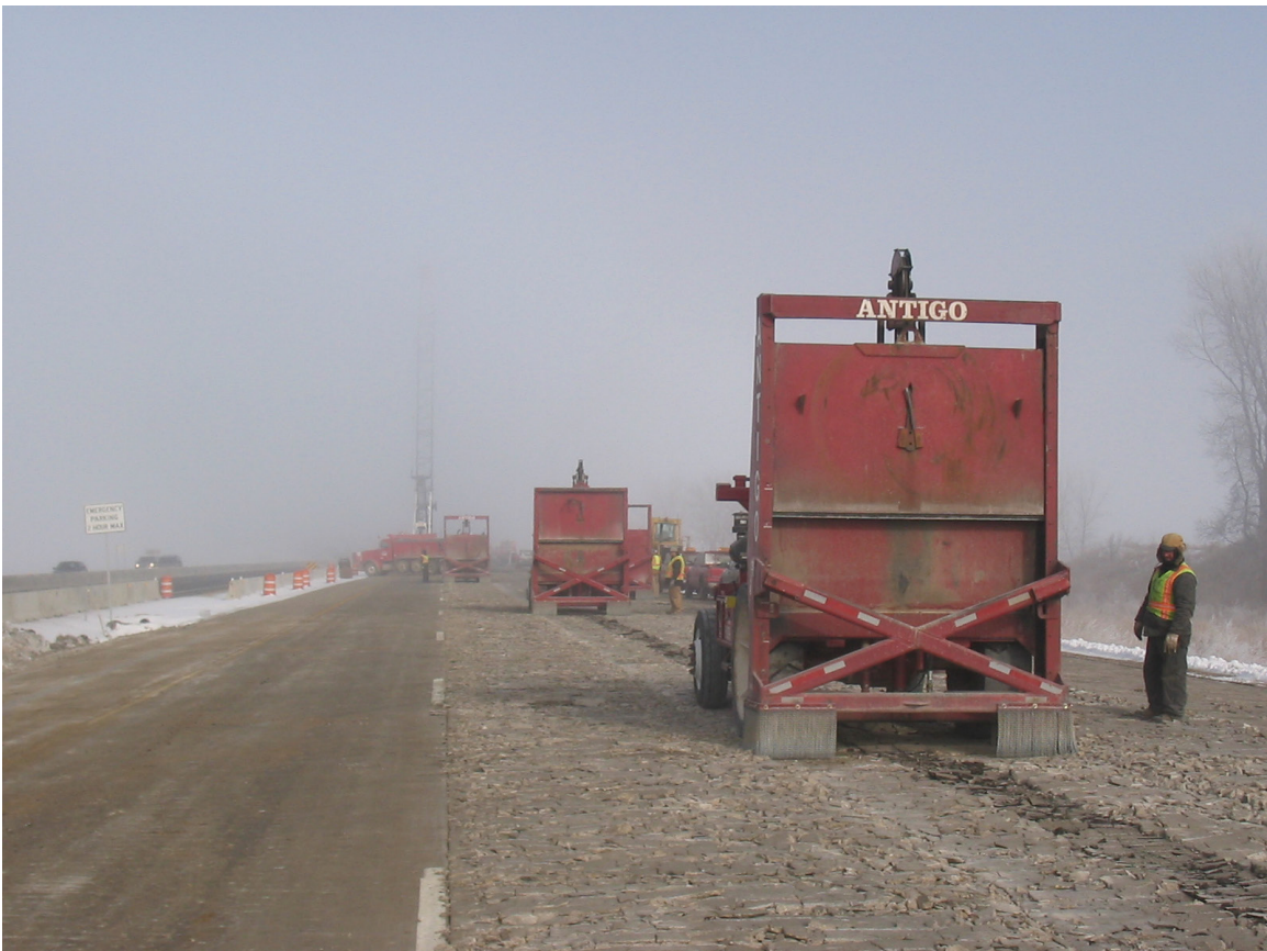
Hammers striking concrete at approximately 6-inch intervals.
