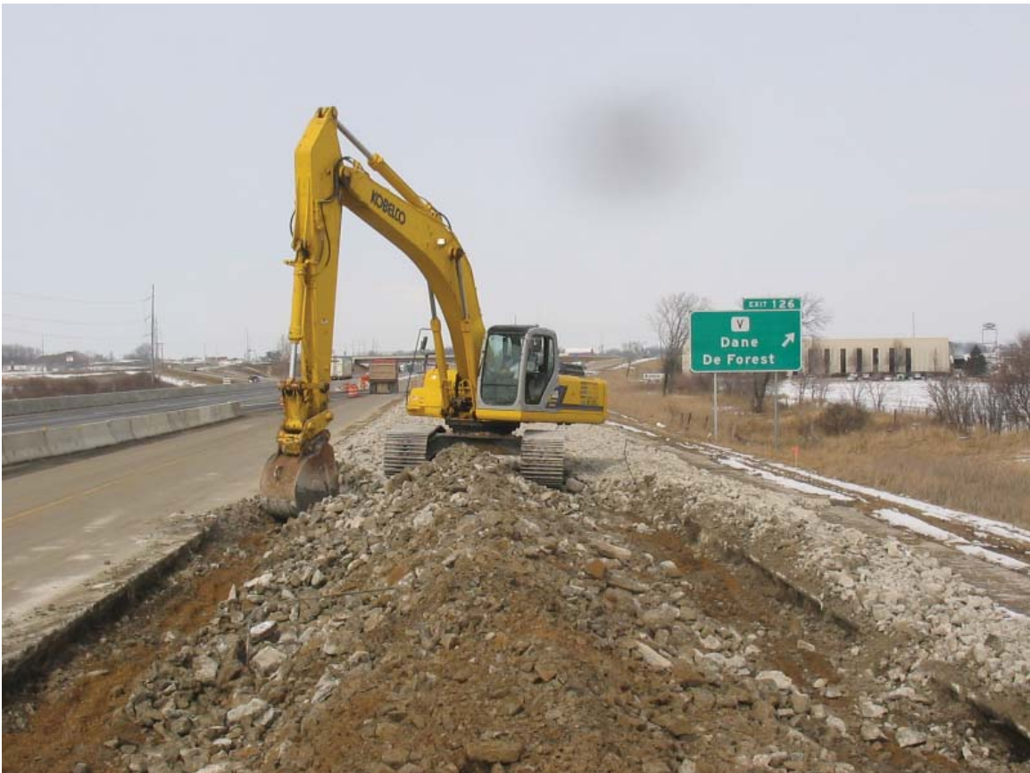
Excavator windrowing broken concrete after reinforcing bar removed.
