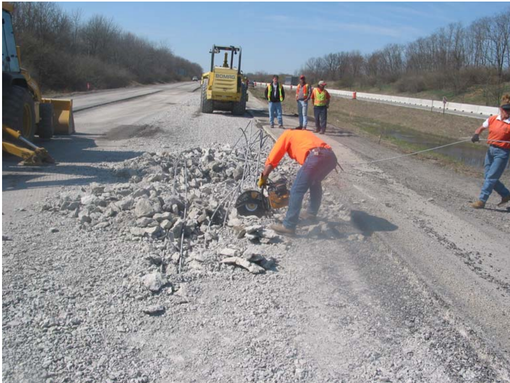
Cutting rebar from test hole to dispose of off site.
