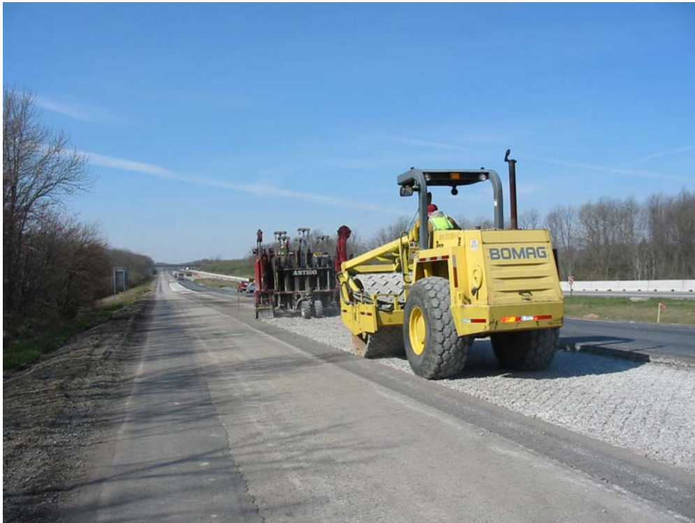
2nd compaction/seating pass with grid roller.
