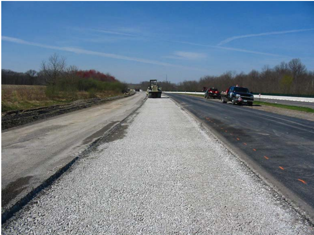
Final surface after compaction/seating - ready to overlay with HMA.
