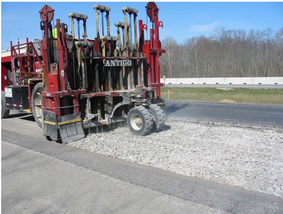
1 lane of existing HMA overlay removed and underlying CRCP rubblized.
