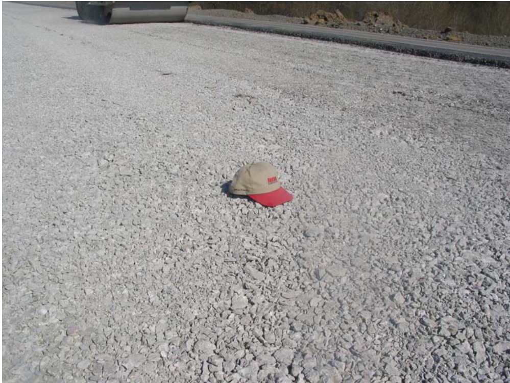
Typical final surface after compaction/seating.
