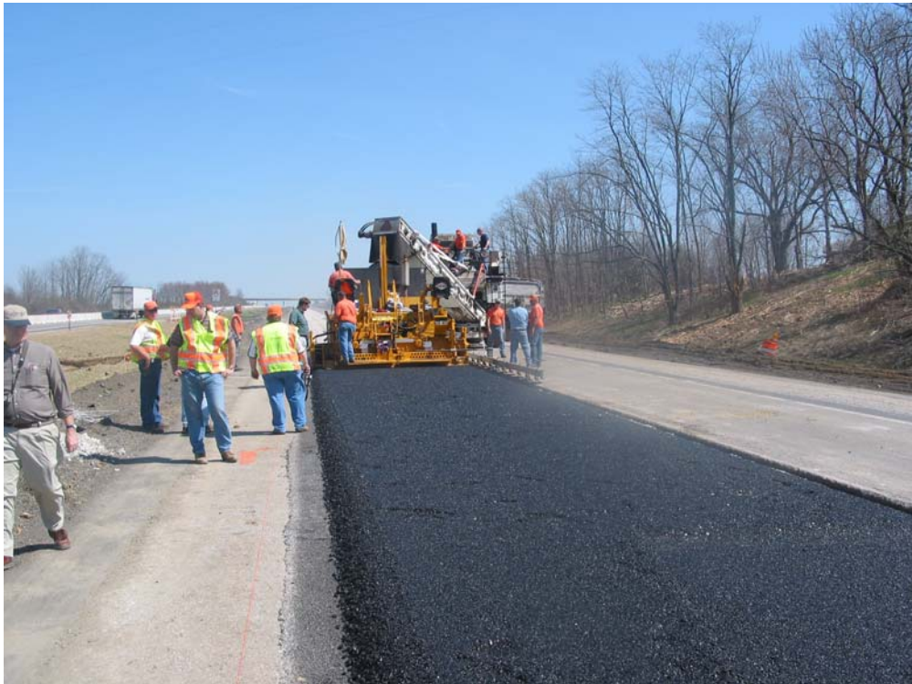
Paving first lift of HMA.
