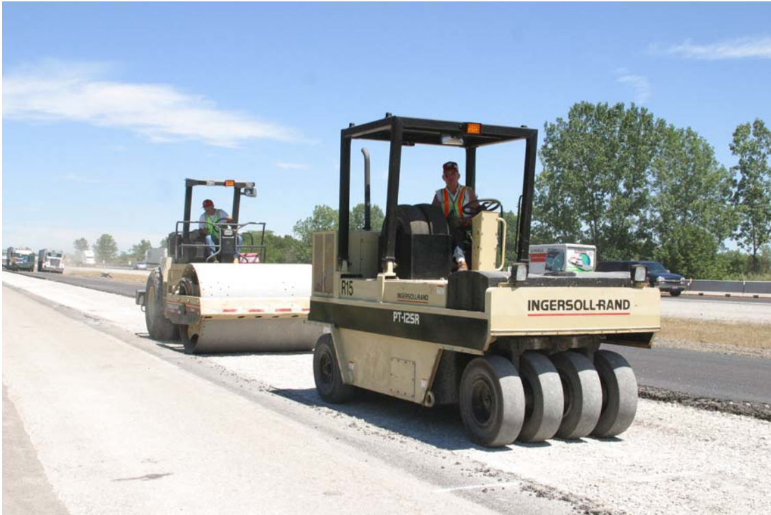
2 passes with PTR and 2 passes with vibratory smooth drum.
