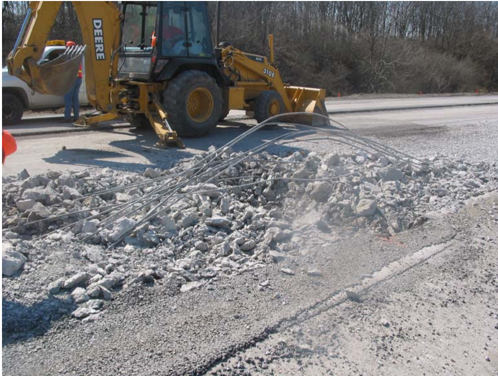
Completed test hole.
