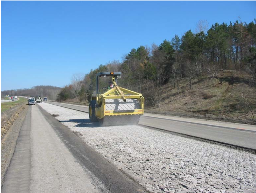
First compaction/seating pass with grid roller.
