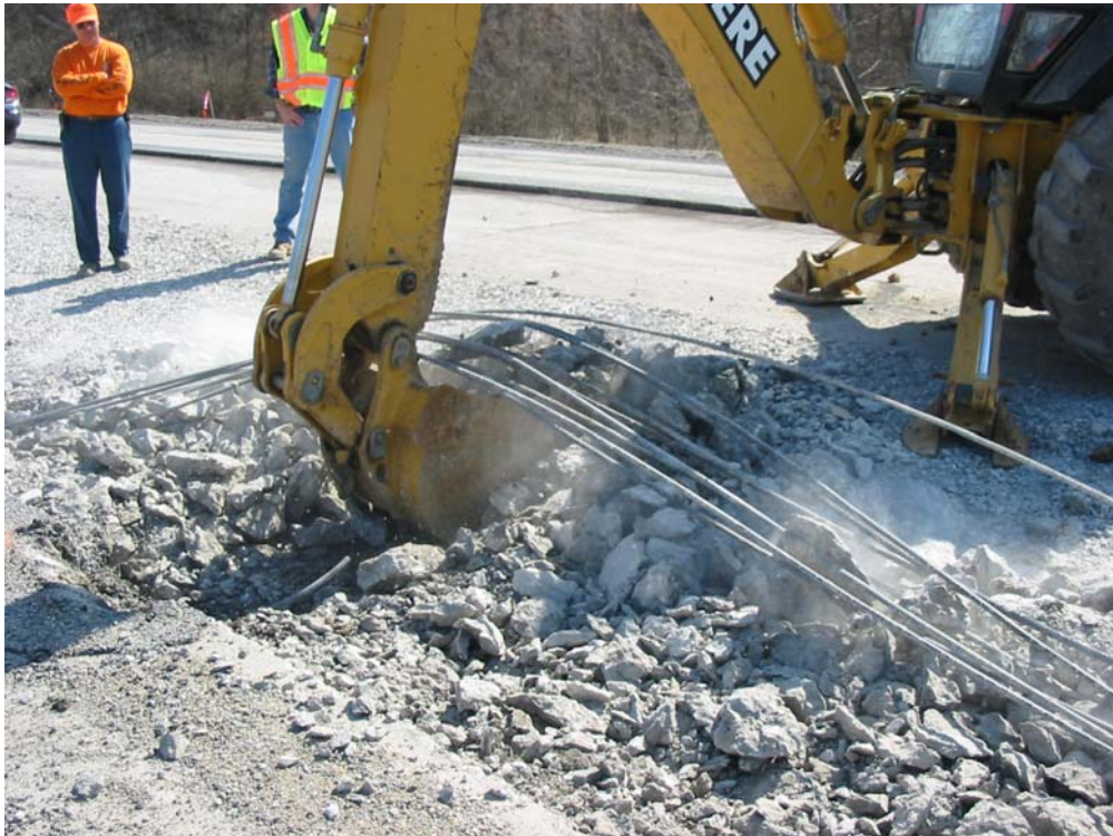
Digging test hole in rubblized CRCP.
