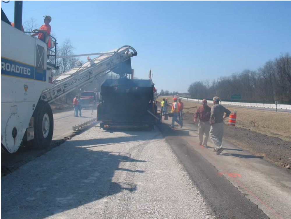
Paving first lift of HMA utilizing an MTD.
