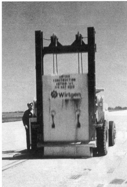
PCC pavement underlying asphalt surface was cracked with a Wirtgen CB700 6-ton guillotine.
