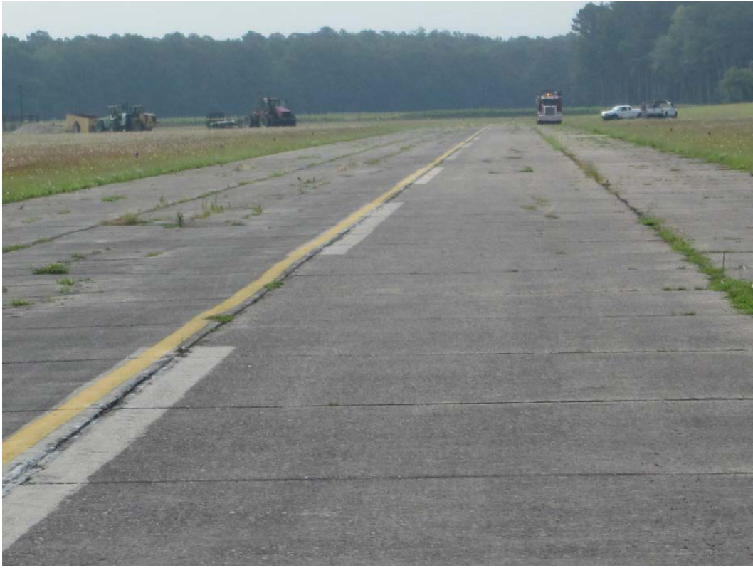
Prior to cracking
