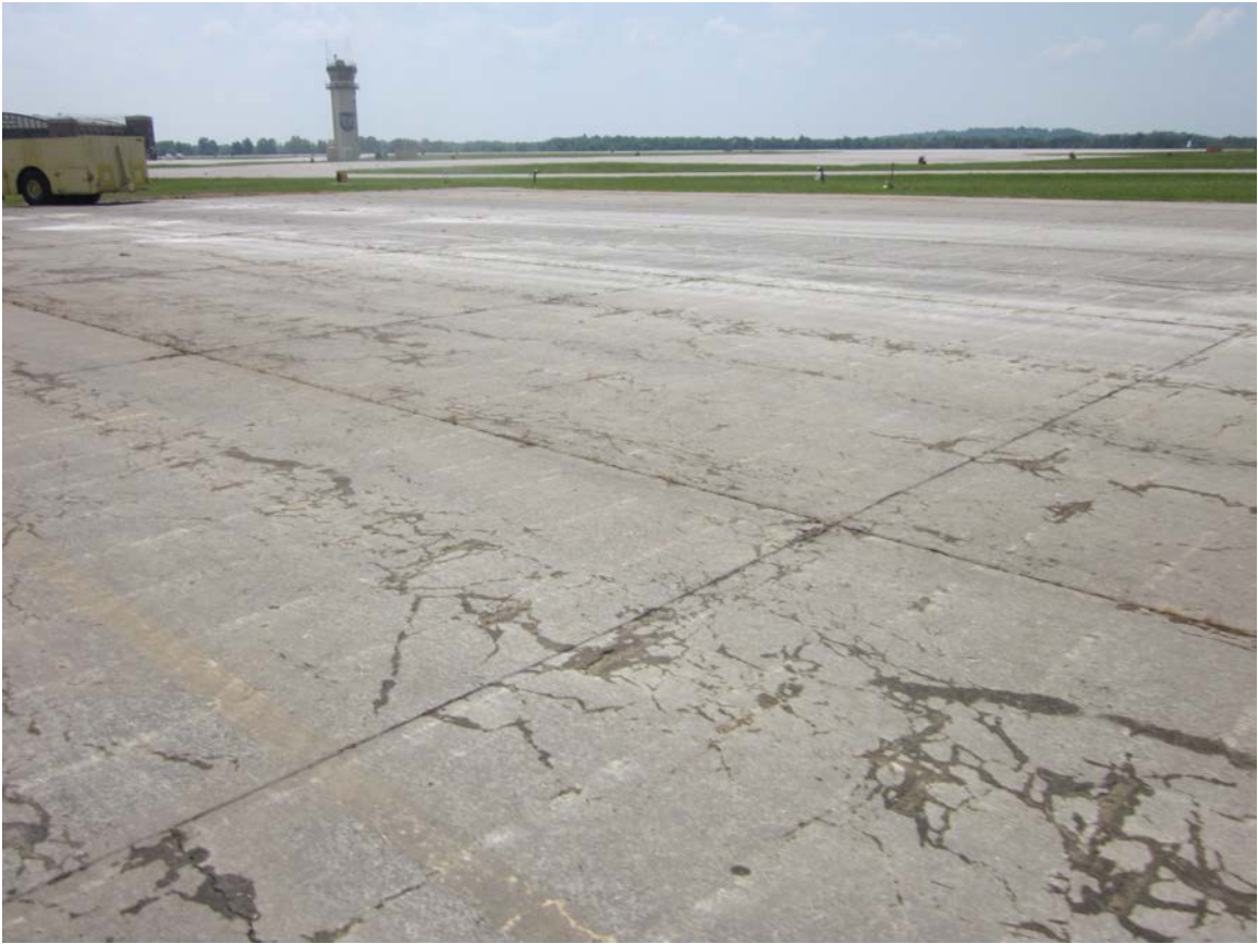
Cracked with T8600 Badger Breaker®
