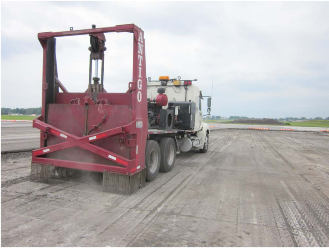
Cracked with T8600 Badger Breaker®
