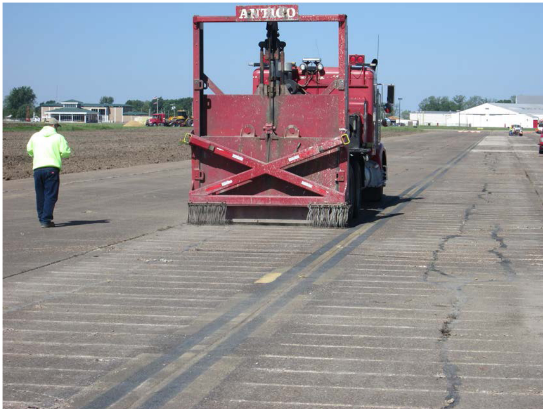
Cracked with T8600 Badger Breaker®
