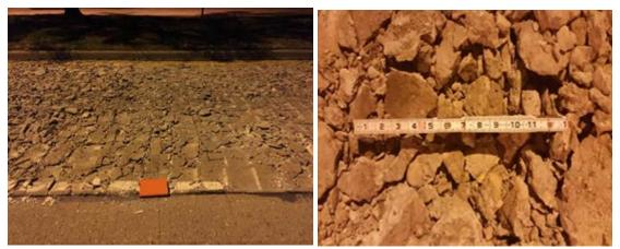
Figure 6. Particle Size After Rubblization (Before Rolling)
