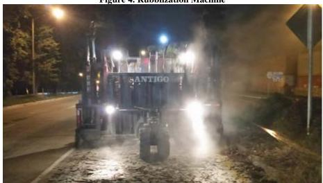
Figure 5. Rubblization Process
