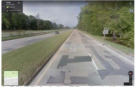
Figure 2. Existing SR 406: CRCP in Poor Condition. CRCP = continuously reinforced concrete pavement.
