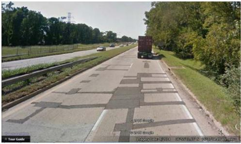
Figure 3. Existing SR 406: CRCP in Poor Condition. CRCP = continuously reinforced concrete pavement.
