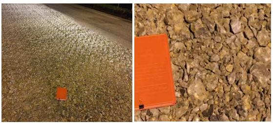
Figure 11. Final Rubblization Surface
