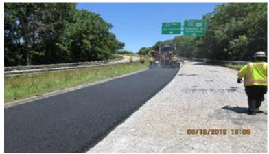
Figure 12. Placement of IM 19.0E Mixture
