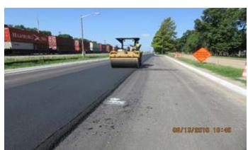
Figure 13. Placement of SM 12.5E Mixture
