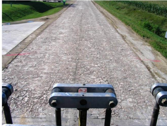
Modified Rubblization—significant spalling
