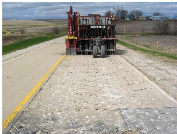
Modified Rubblization—significant spalling
