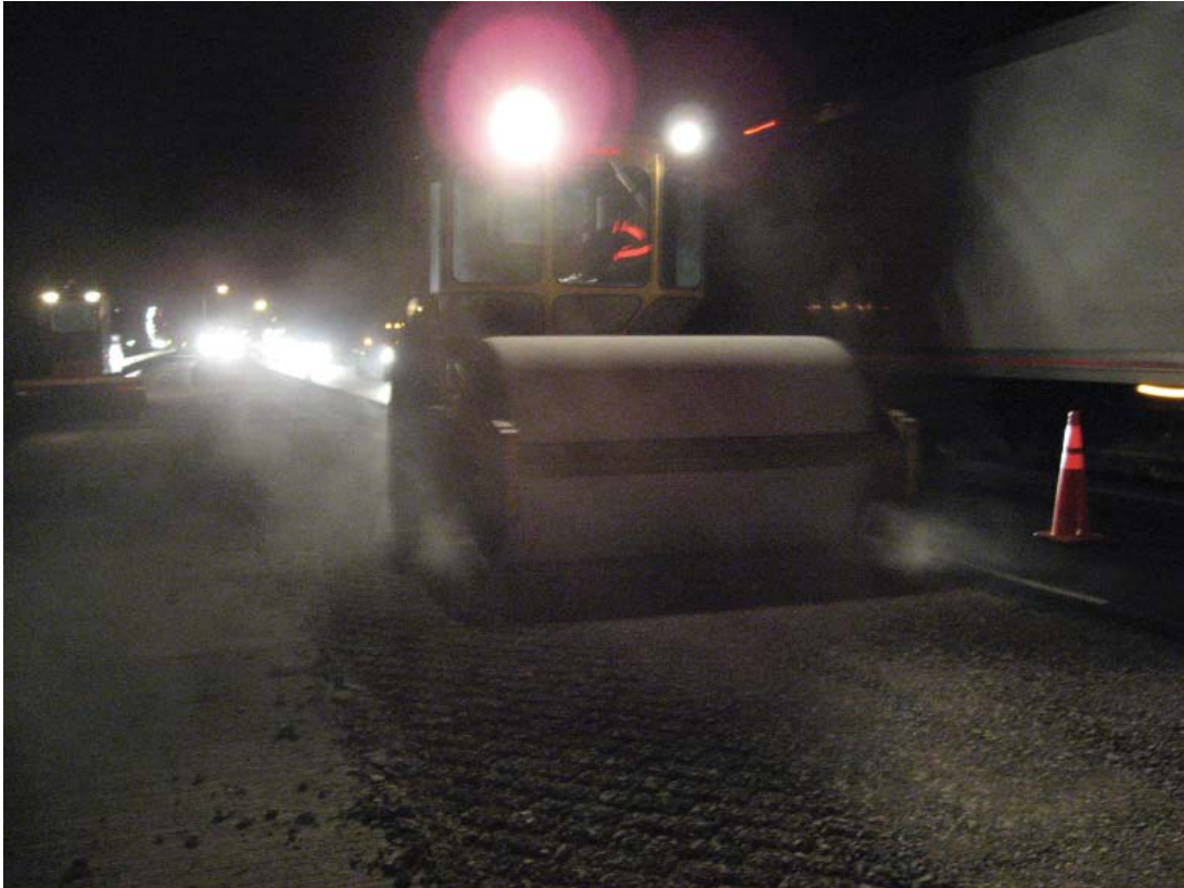
Smooth drum roller completing the rolling.
