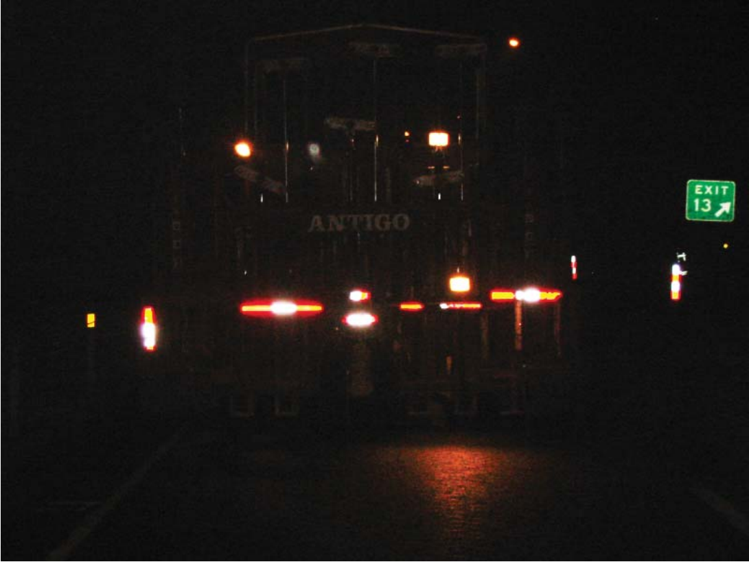
MHB Badger Breaker® rubblizing at night.
