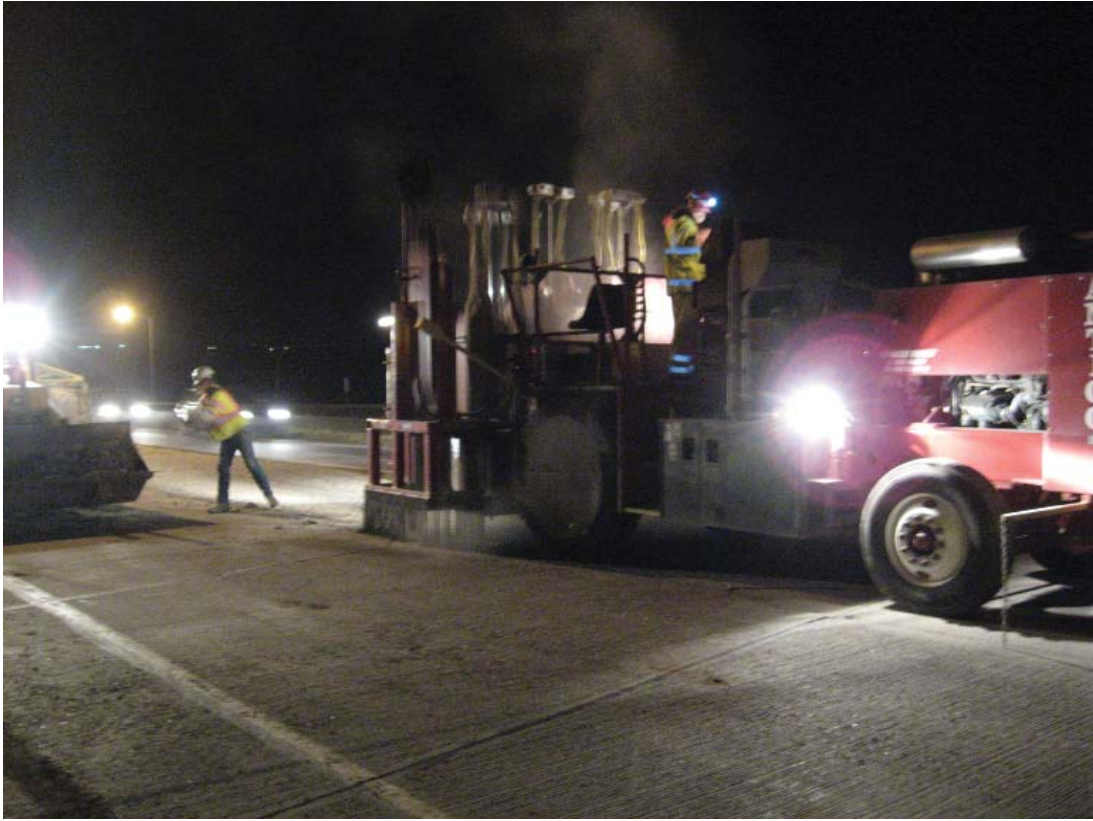
MHB rubblizing followed by crew removing miscellaneous joint sealant and patching.
