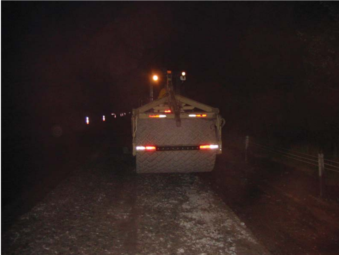
Grid roller pulverizes surface particles and begins compaction of rubblized concrete.
