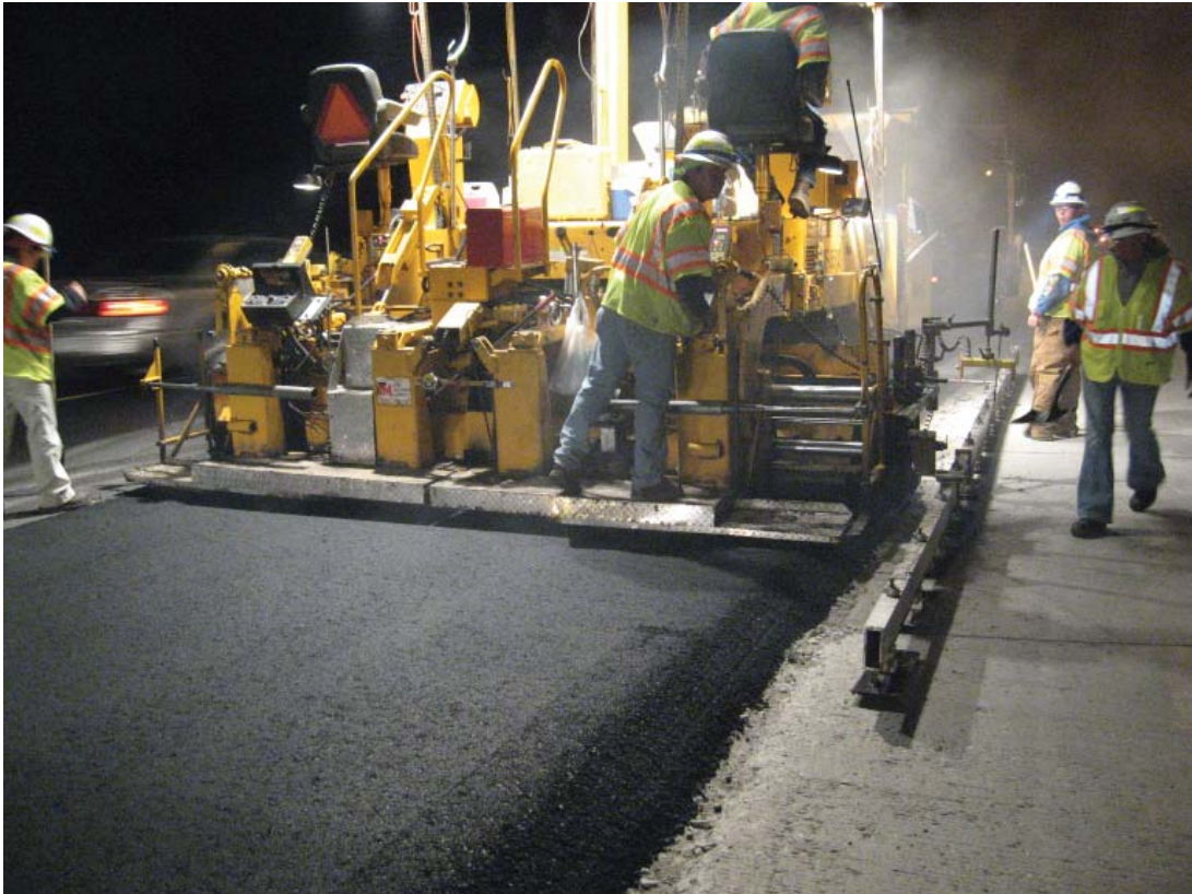
Paving first lift of asphalt overlay.
