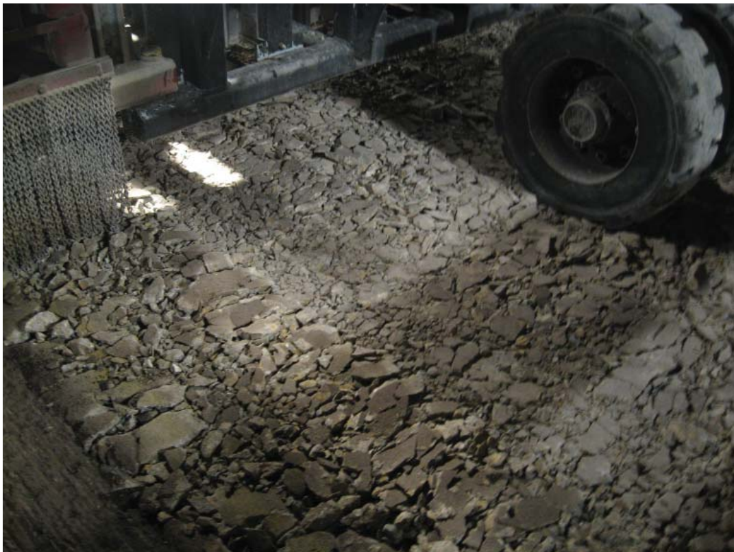
Close up of rubblized surface prior to rolling.
