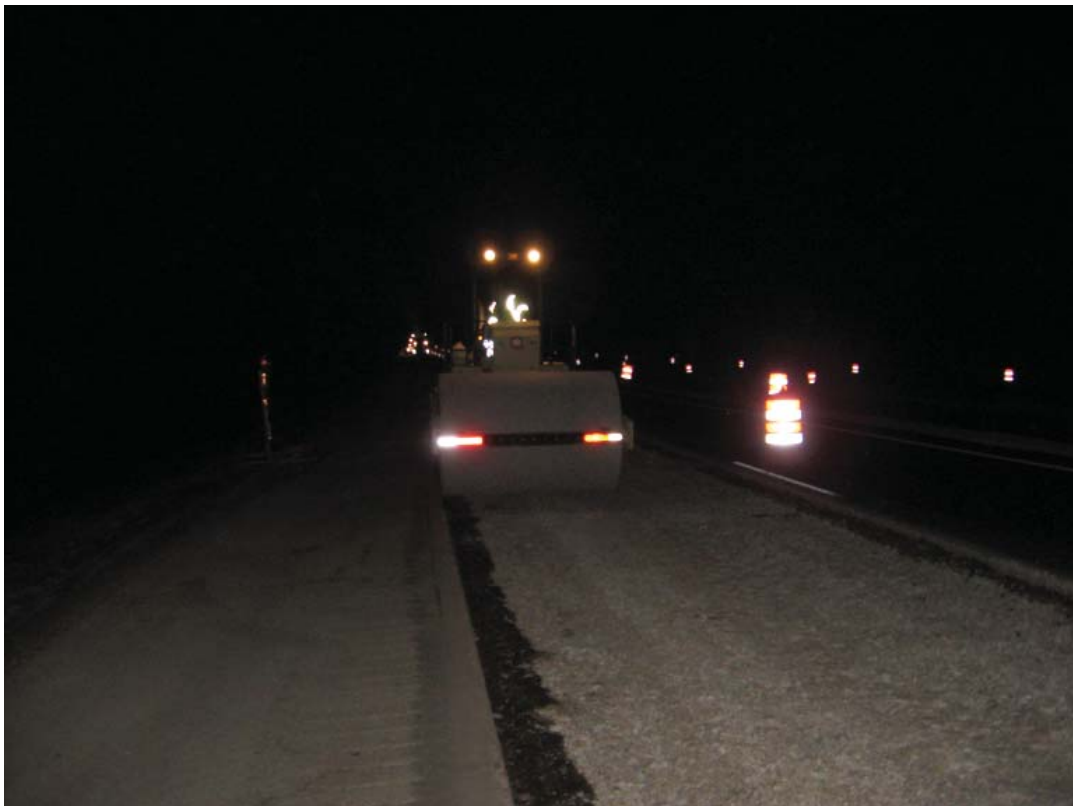
Smooth drum roller completing the rolling.
