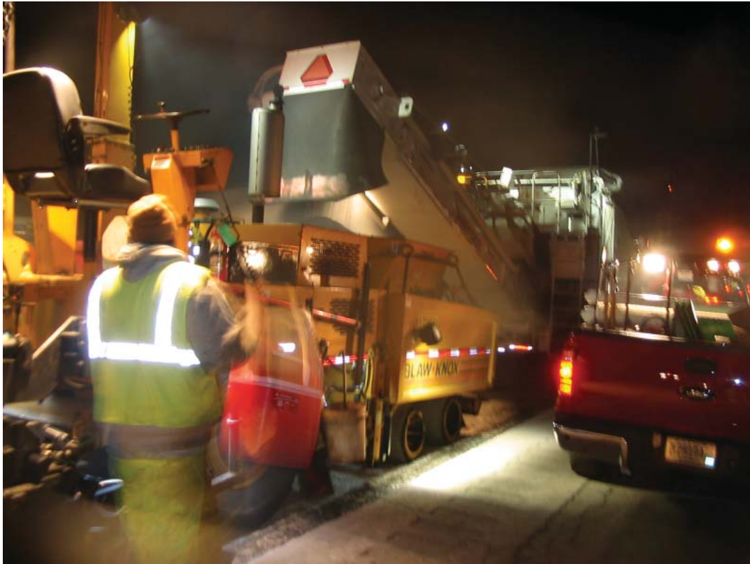
Paving asphalt overlay using Material Transfer Vehicle (shuttle buggy).
