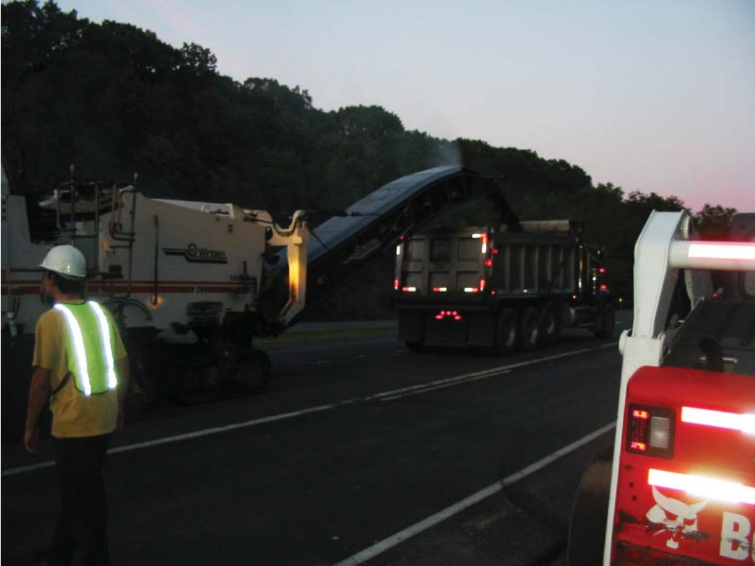
Milling off existing asphalt overlay in one lane.
