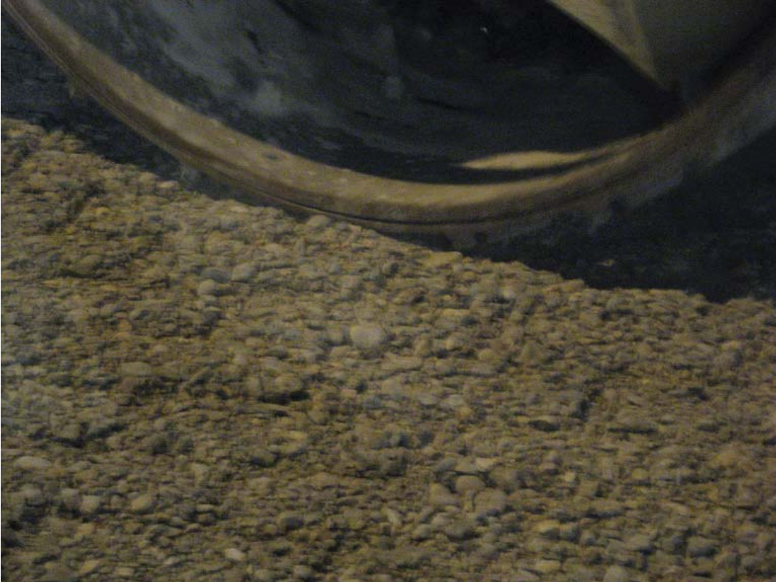
Close up of grid roller pulverizing surface particles.
