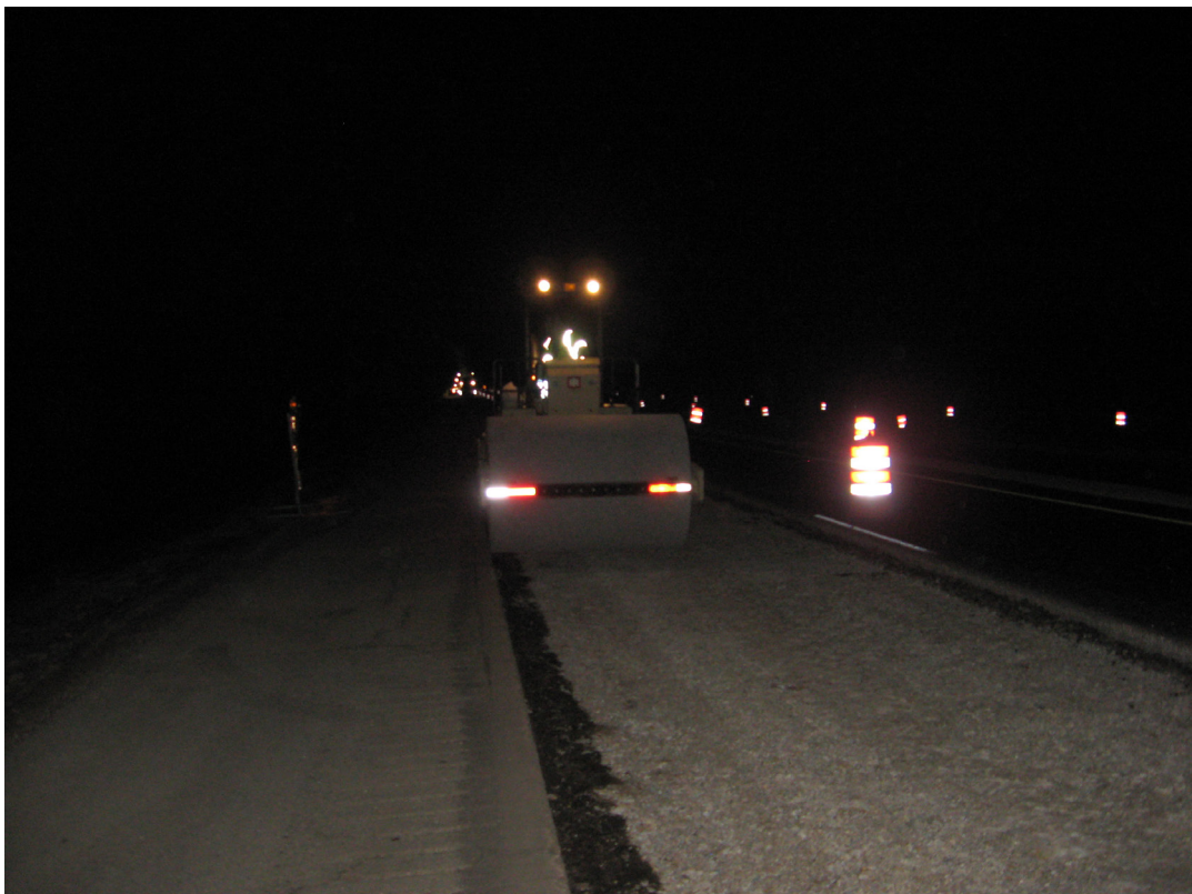
Smooth drum roller completing the rolling.
