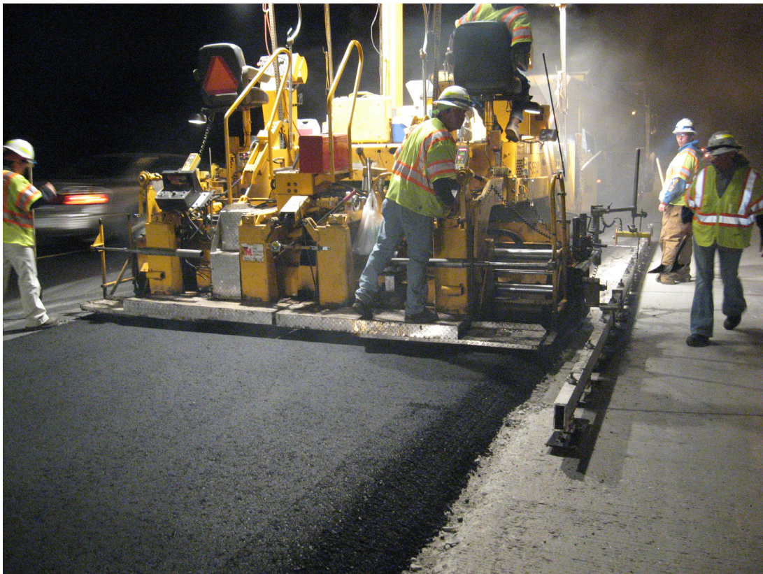
Paving first lift of asphalt overlay.
