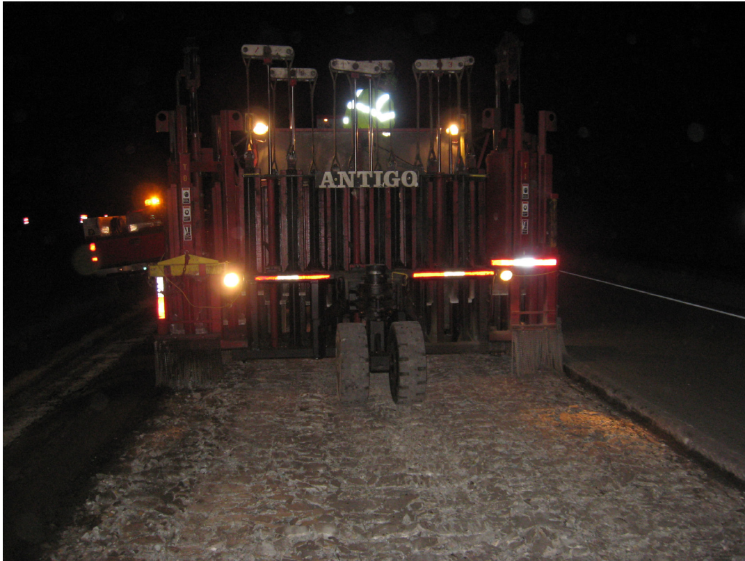
MHB Badger Breaker® rubblizing at night after existing asphalt overlay milled off. Note existing asphalt overlay in place on right lane.
