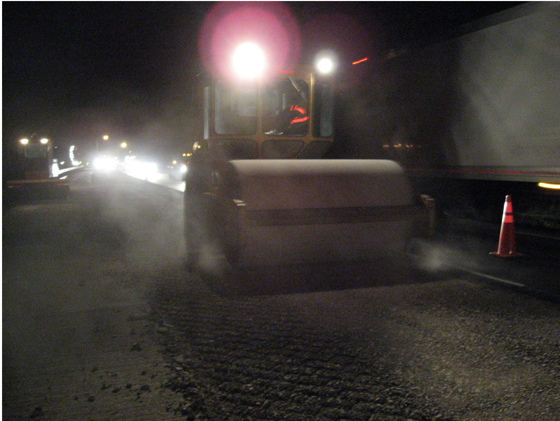
Smooth drum roller completing the rolling.
