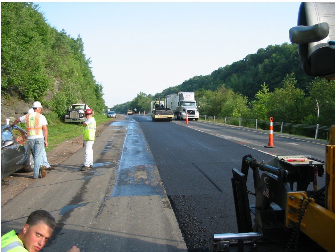
Finishing paving early next morning. Note that first lift of new asphalt overlay matches up with existing overlay on adjacent lane.
