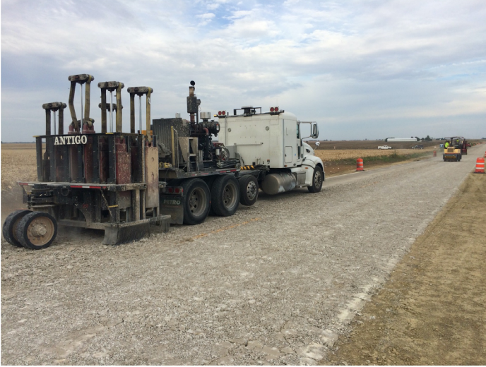
An Antigo multi-head breaker rubblizes the original concrete section.
