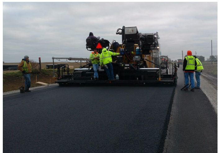
Paving full-width to eliminate longitudinal joint.
