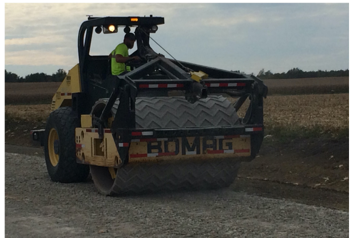
Z-grid roller used to compact the rubblized section.
