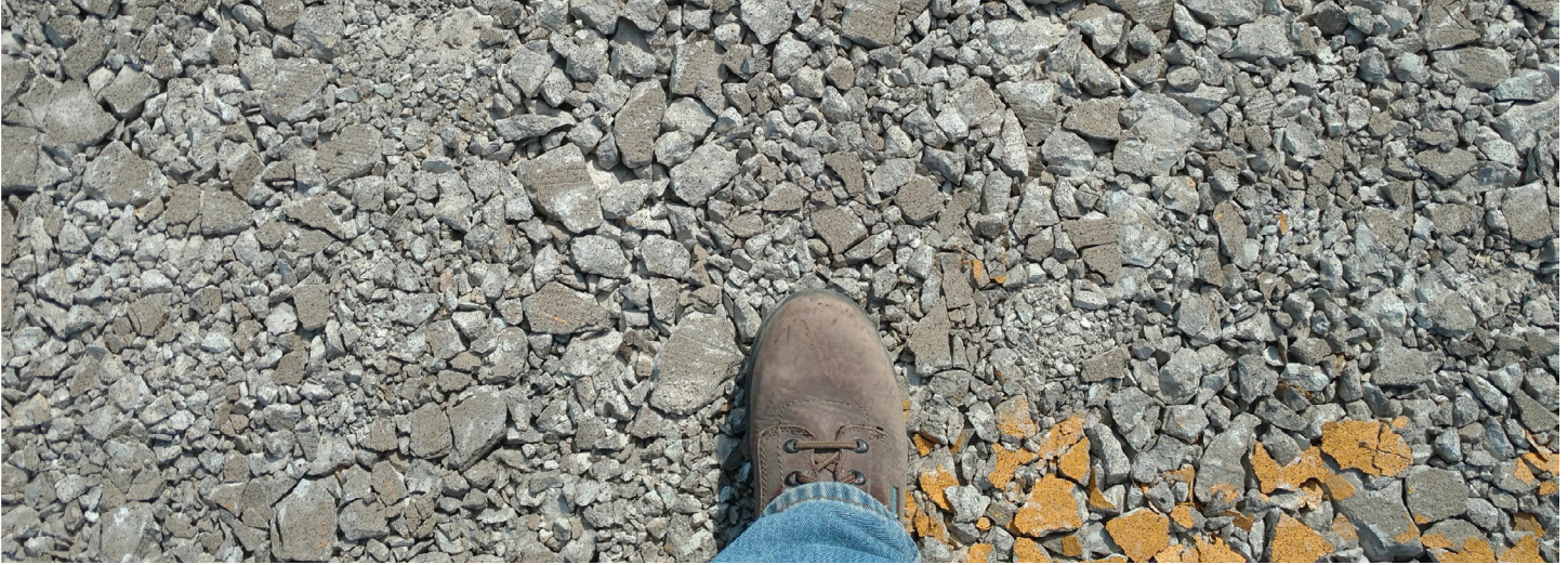
Concrete surface after rubblization and compaction prior to HMA overlay.
