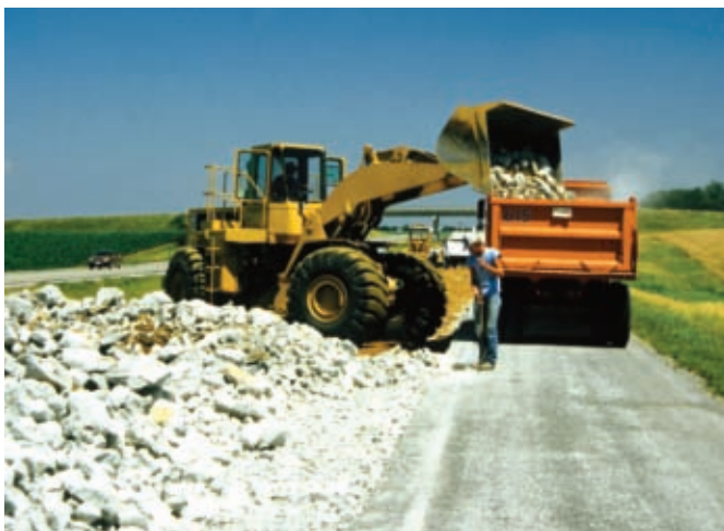
Figure 12. Removal and transport of broken pavement fragments using end loader and dump truck.
