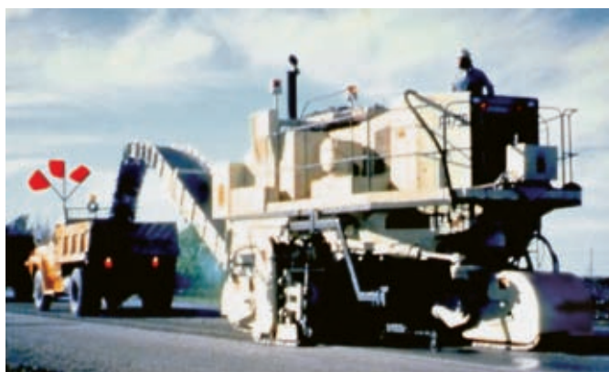
Figure 4. Asphalt pavement surface removal using cold milling machine (Photo credit: National Highway Institute).
