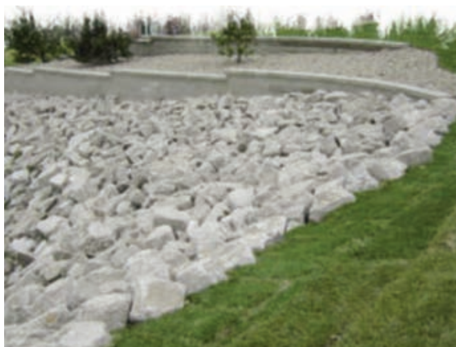
Figure 20. Photo of recycled concrete pavement used as “rip-rap” for erosion control (Photo credit: Blessing Construction, Kearney, NE).
