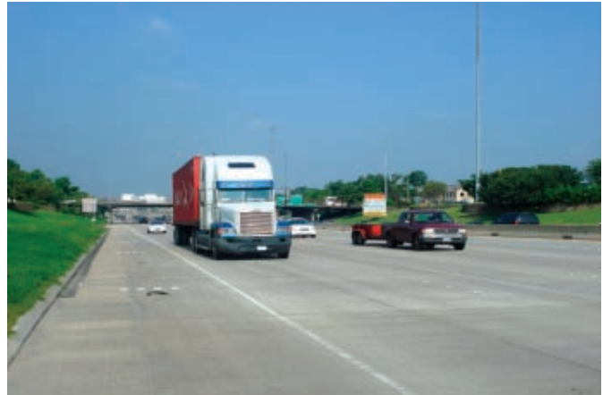
Figure 25. Photo of I-10 RCA CRCP near Houston, Texas.
