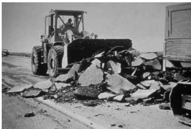
Figure 5. Asphalt pavement surface removal using heavy scraper and end loader (Photo credit: National Highway Institute).
