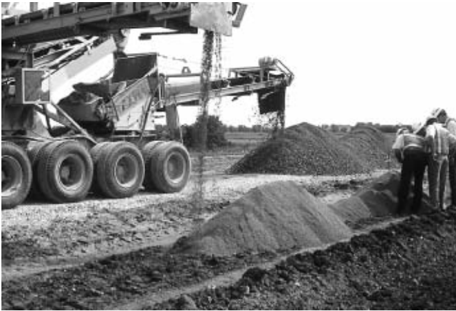
Figure 17. In-place recycling of an existing concrete pavement with the coarse and fine RCA being separated as part of the process (Photo credit: Iowa DOT).
