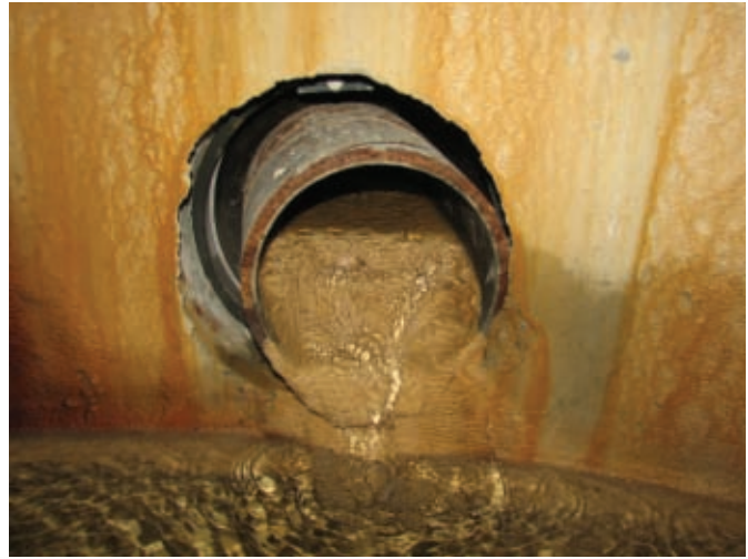
Figure 27. Photo of extreme (atypical) case of calcium carbonate precipitate in a drainage outlet (Photo credit: Richard Proszek, City of Seattle Materials Laboratory).
