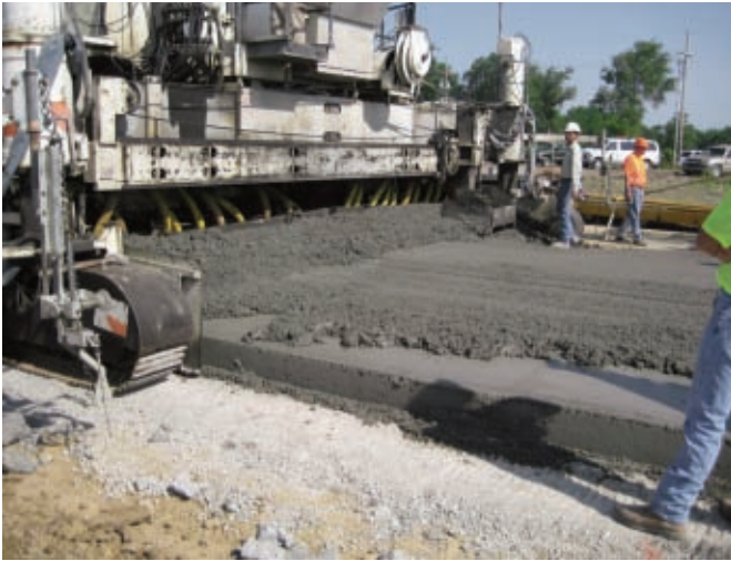
Figure 28. Two-course concrete pavement construction; this photo was taken after the first lift was spread and consolidated and the second lift was spread, but before the second lift was slipformed, showing the second slipform paving machine and top lift (Photo credit: Missouri/Kansas Chapter, ACPA).
