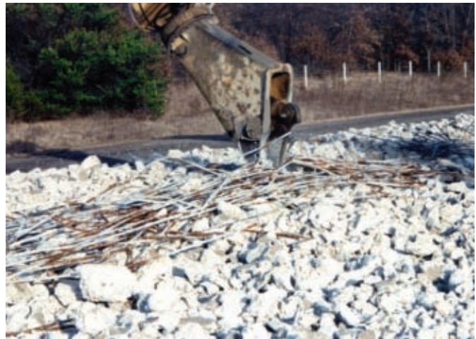
Figure 13. Removal of reinforcing steel on the job site or after crushing.
