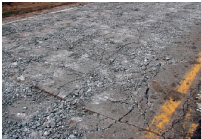
Figure 10. Typical crack pattern for broken concrete pavement prior to removal.
