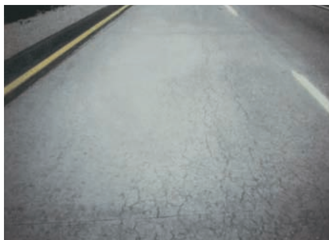
Figure 22. Photo of I-80 in Wyoming prior to recycling. Note ASR damage throughout (Photo credit: Wyoming DOT).
