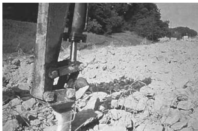
Figure 11. “Rhino horn” for use in loosening broken pavement fragments.
