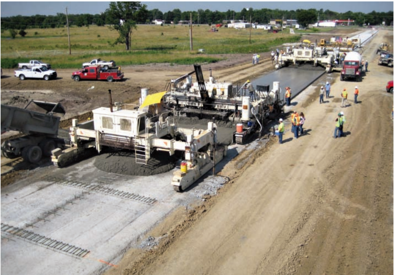
Figure 29. Two lift construction of a portion of I-70 in Salina, KS in 2008; note that in the paving train there are two combinations of placers and slipform pavers, one for each lift, followed by texturing and curing machines (Photo credit: Missouri/Kansas Chapter, ACPA).
