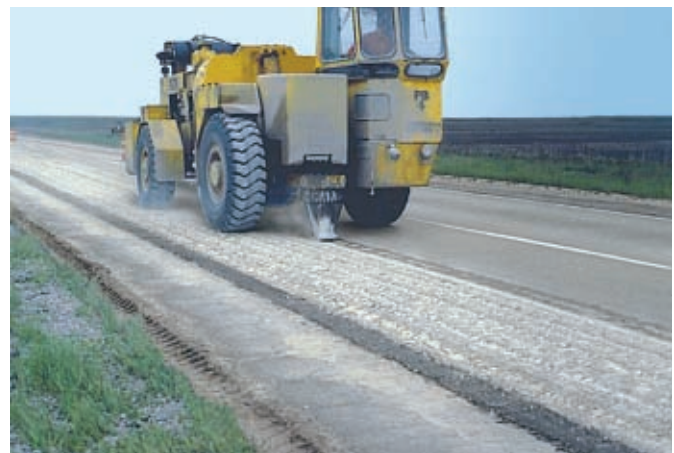
Figure 9. Vibrating beam pavement breaker.
