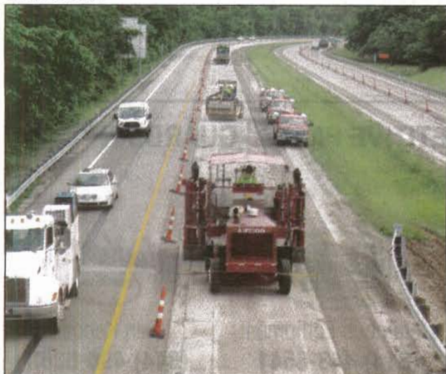
Antigo Construction's multi-head breakers were used in virtually all of the concrete breaking activities on the WVDOH projects.
