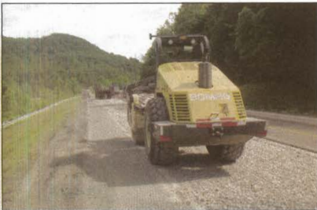
The cost of rubblization and new asphalt is roughly $143,000 per mile, representing a savings of approximately 13 to 28 percent over traditional remove-and-replace paving.
