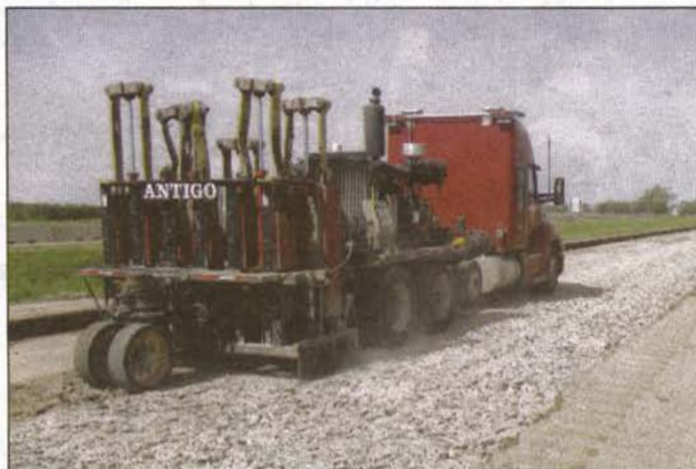
Rubblizing breaks the bonds between any reinforcing steel and the concrete, eliminating slab movement and decreasing the chance of future reflective cracking.
