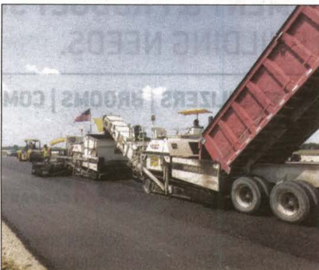
Contractors place an asphalt layer on top of the base, creating a new road with years of service for the driving public.
