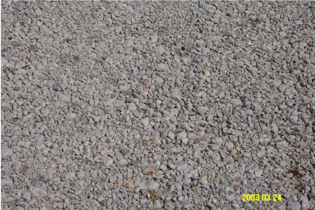
FIGURE 7 The final rubblized and compacted PCC surface.
