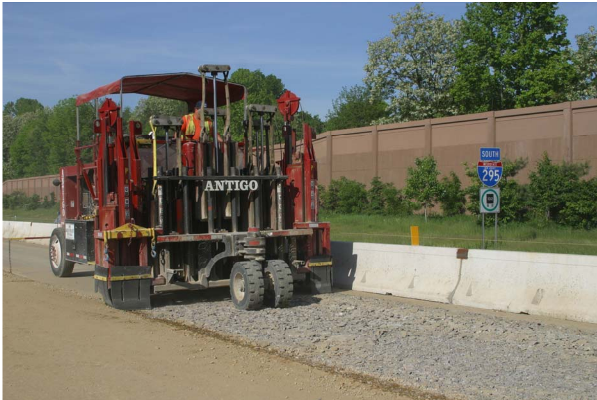
FIGURE 4 The MHB operating working close to a barrier.
