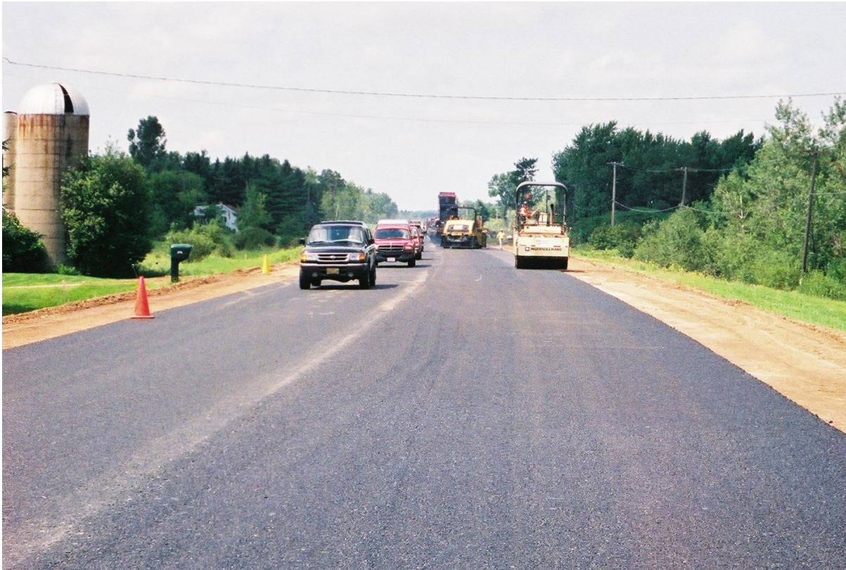
Paving the first lift of asphalt on the second lane
