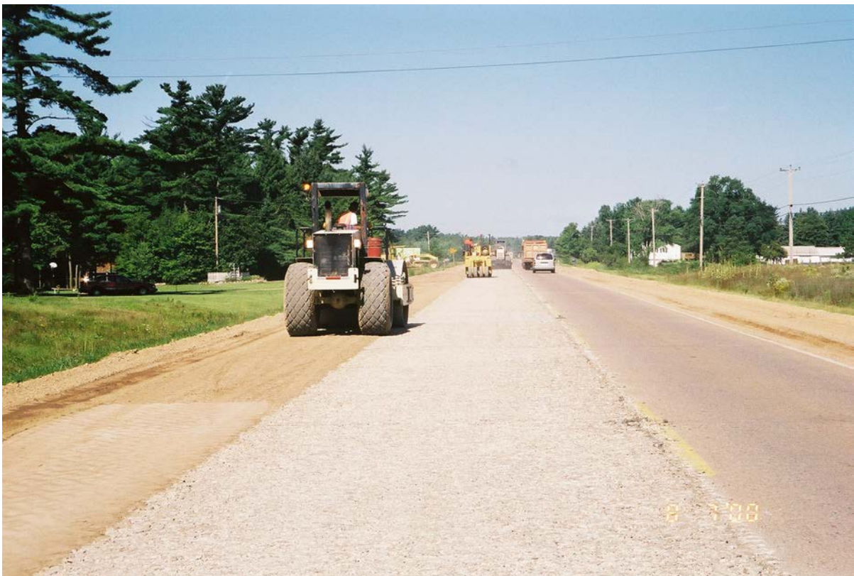
Rolling and seating the first lane
