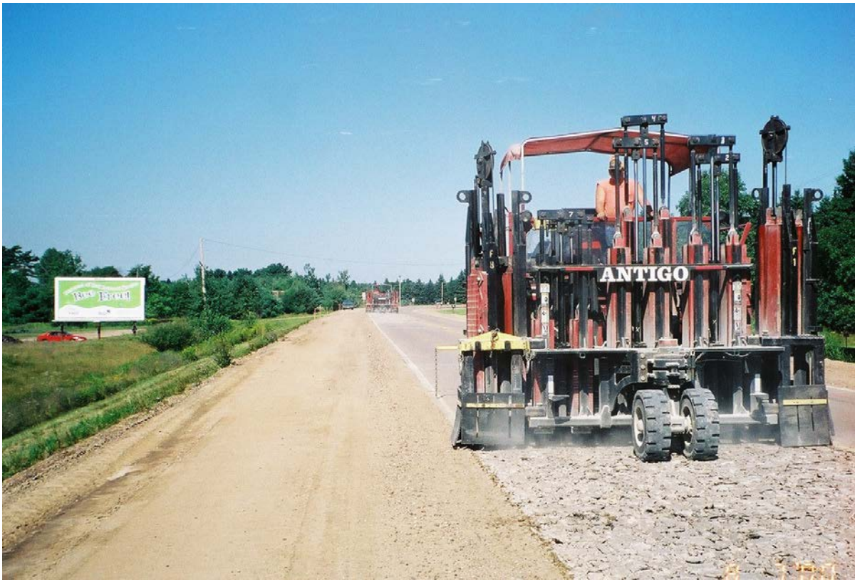
Rubblizing the first lane in the morning
