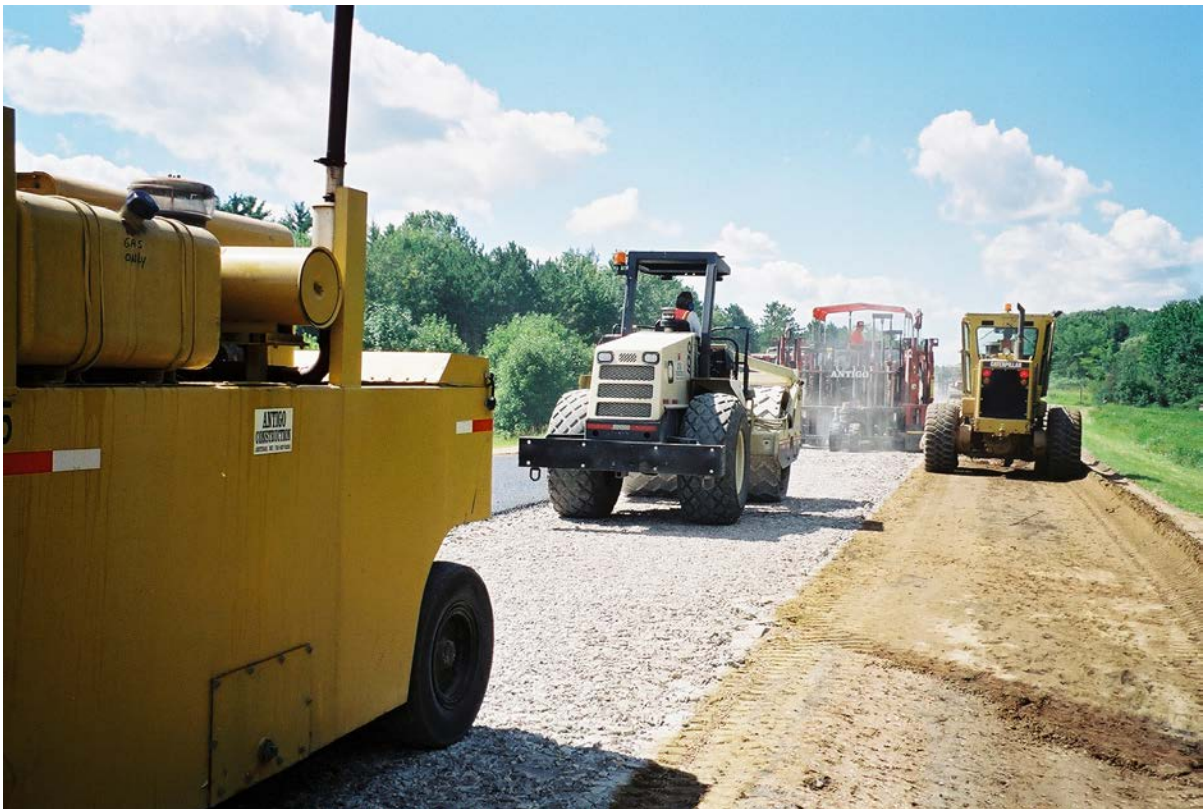
Rolling and seating the second lane
