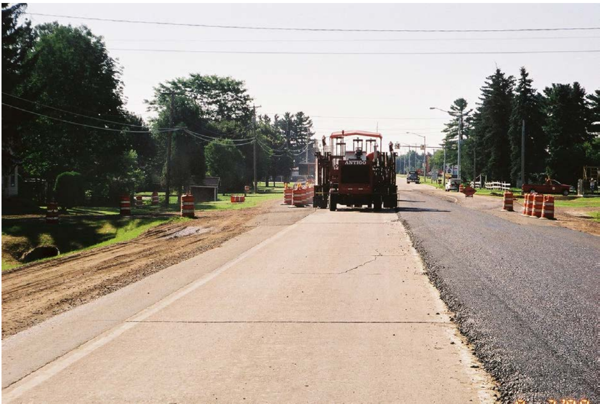
Rubblizing the second lane in the afternoon
