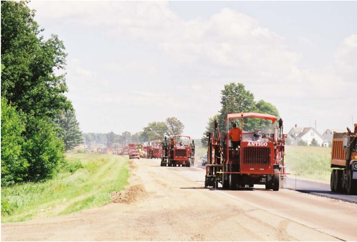
Rubblizing the second lane in the afternoon
