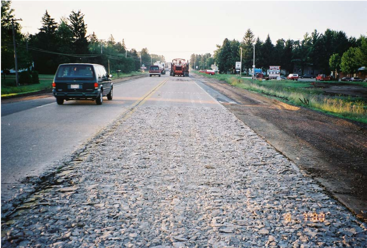
Rubblizing the first lane in the morning
