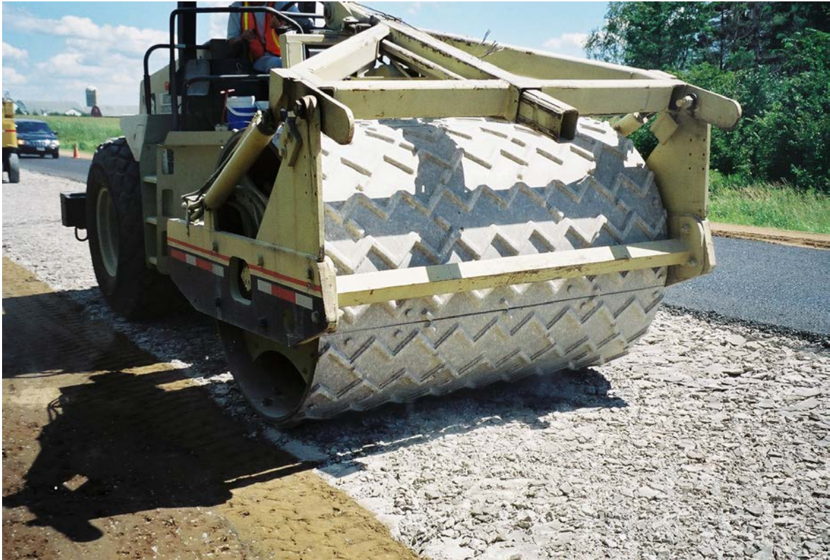
Rolling and seating the second lane
