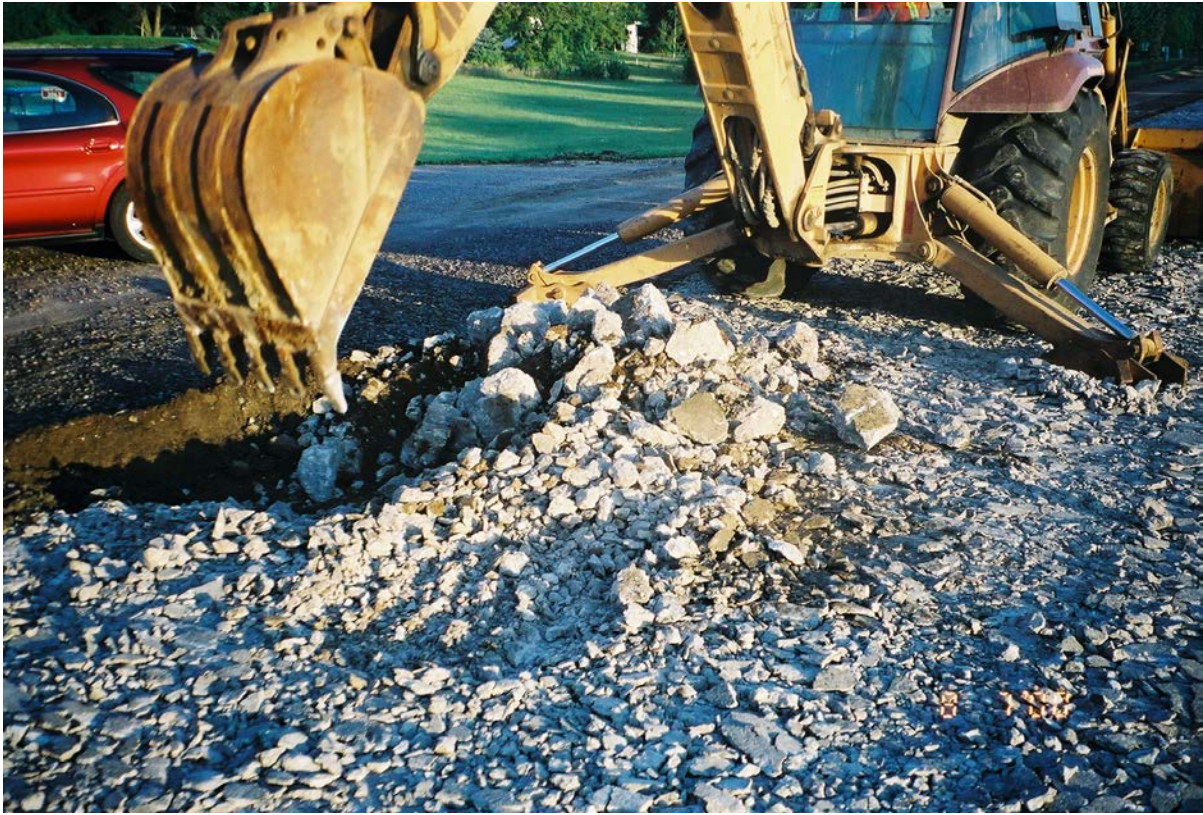
Excavating a test hole the first morning
