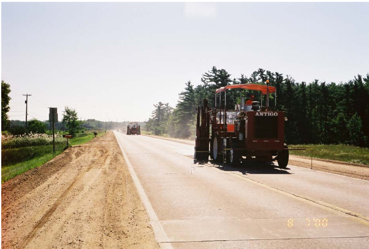
Rubblizing the first lane in the morning
