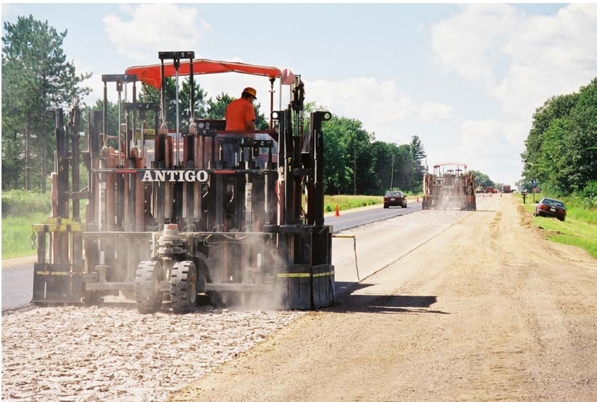
Rubblizing the second lane in the afternoon
