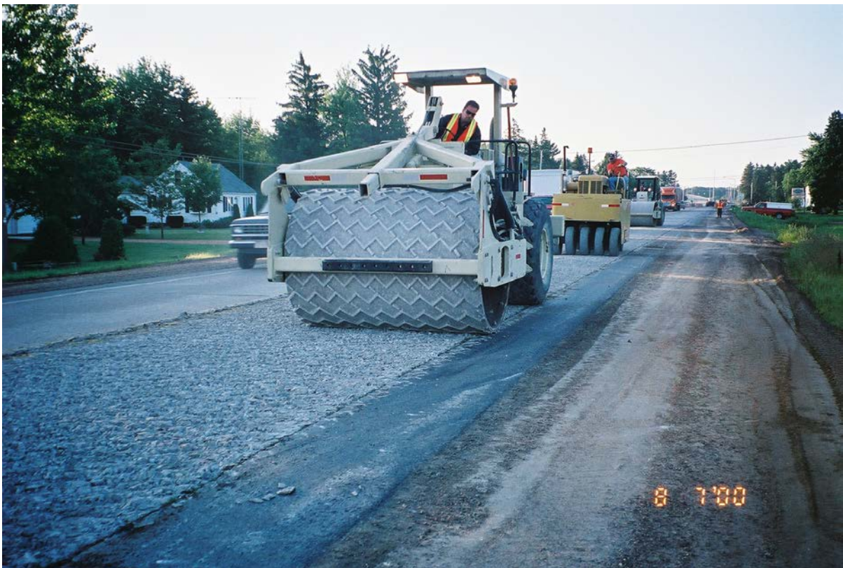
Rolling and seating the first lane
