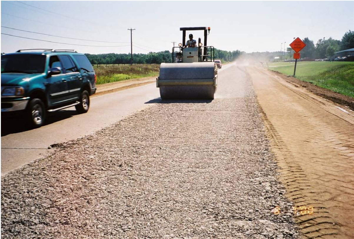
Rolling and seating the first lane
