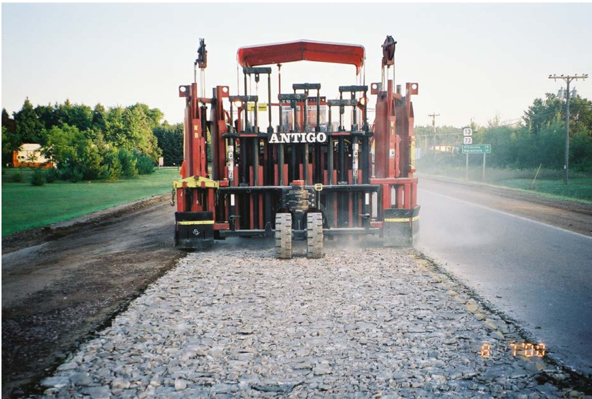
Rubblizing the first lane in the morning
