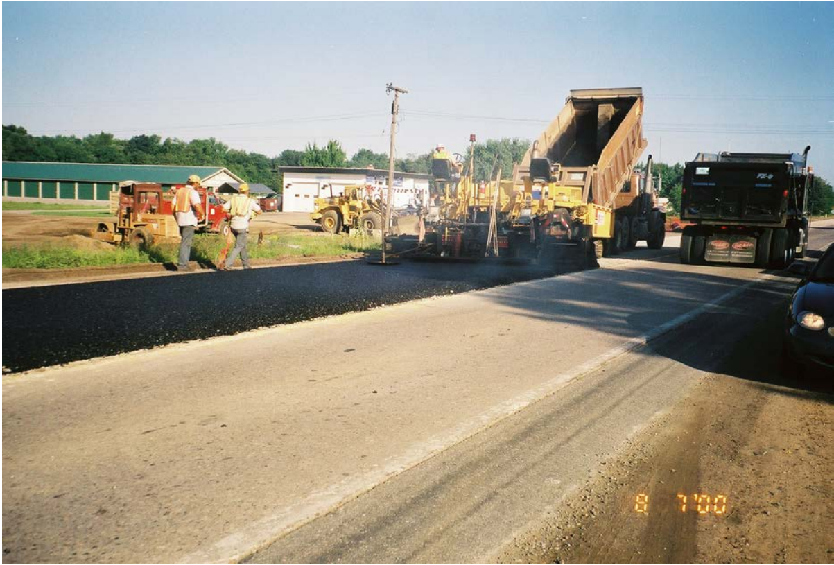
Paving the first lift of asphalt on the first lane
