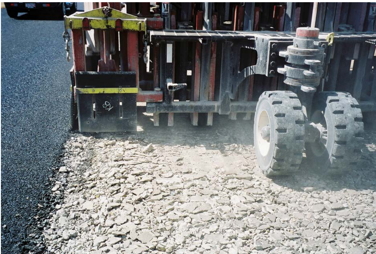
Rubblizing the second lane in the afternoon
