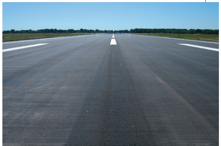
Rubblization and repaving completed at Selfridge Air National Guard Base in Michigan.
