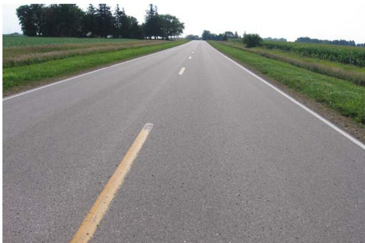
**Fig. 4.** Picture of distress-free HMA surface on rubblized PCC (test section no. 4: C23 in Franklin county)
