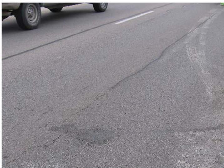
**Fig. 5.** Picture of Longitudinal crack on HMA surface over rubblized PCC (test section no. 6: IA141 in Polk county)
