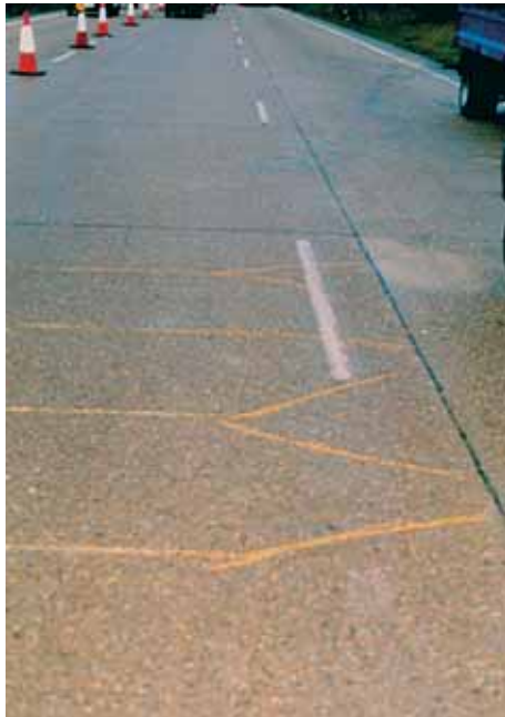
Plate 6.4 Typical satisfactory crack patterns at the edge of the slab
