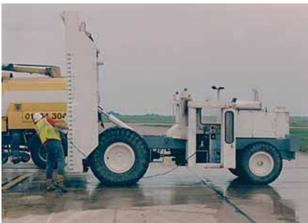
Plate 3.2 Badger Breaker initiating a slab halving crack on a taxiway
