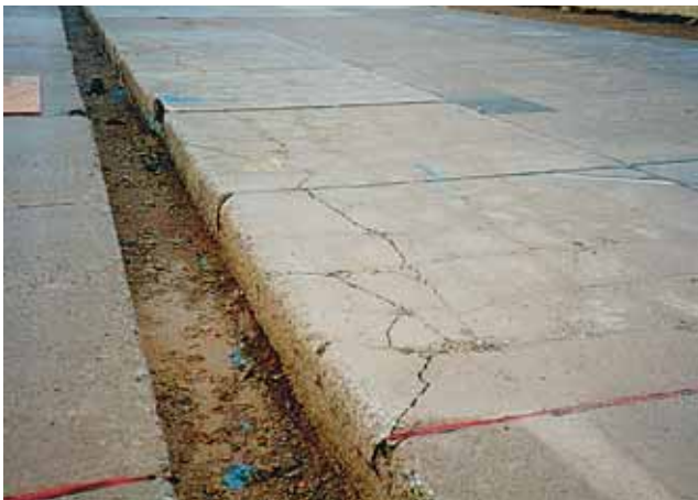
Plate 6.1 Cracking at excavated trench
