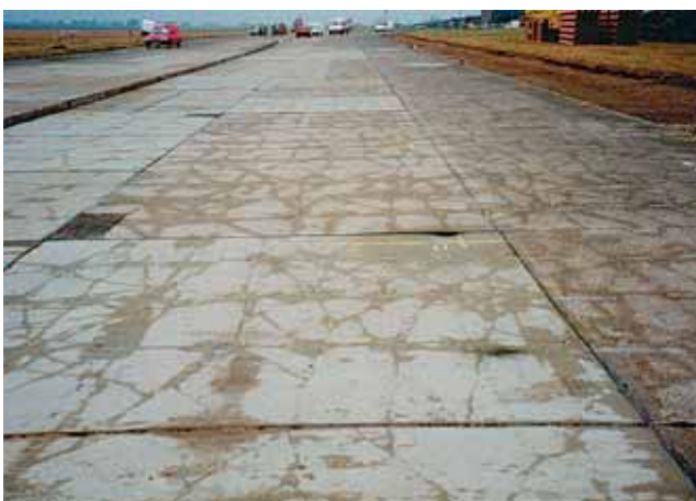
Plate 6.5 Unsatisfactory ‘crazy paving’ crack pattern
