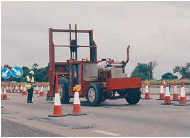
Plate 3.1 Badger Breaker working on a motorway
