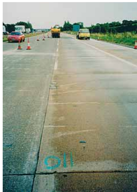
Plate 6.3 Transverse cracking
