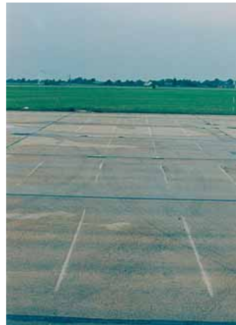
Plate 6.12 Good alignment of cracking across width of taxiway
