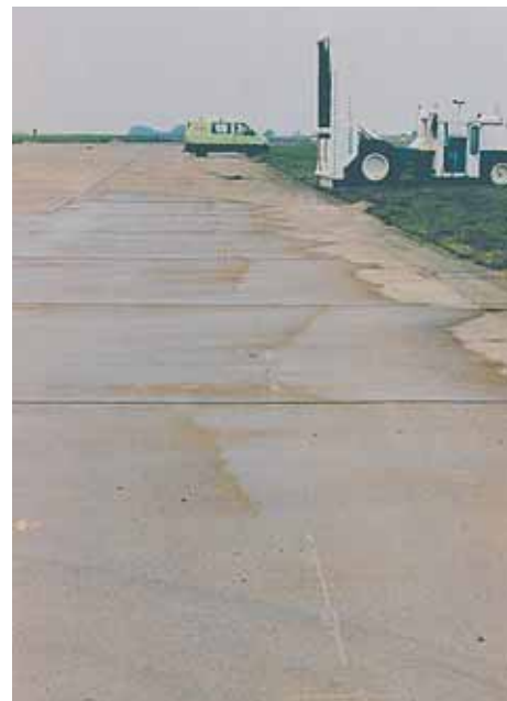
Plate 6.6 Halving large slabs
