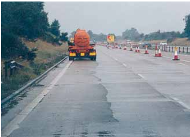
Plate 6.7 Longitudinal cracking due to internal stress or weakness within the slabs
