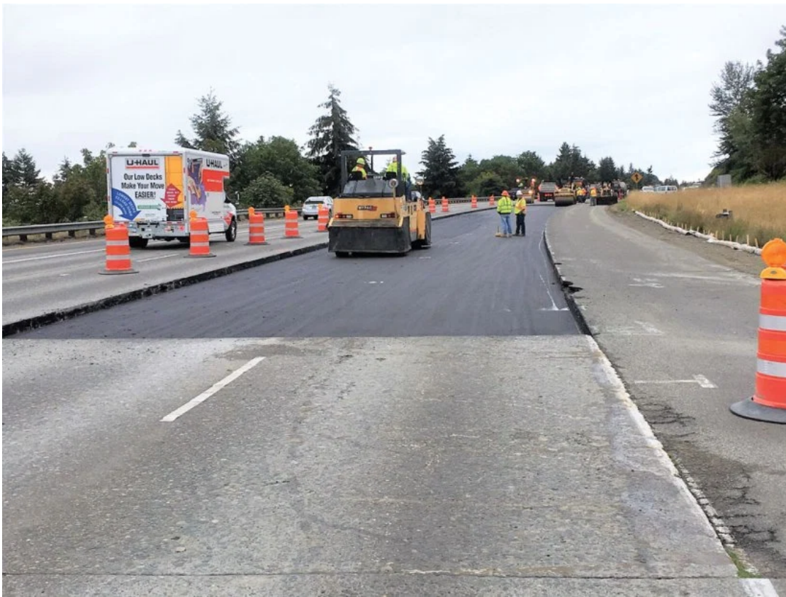
A 35-ton pneumatic roller reseats concrete panels on I-5.
