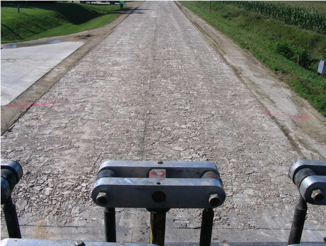
Example of more significant spalling.
