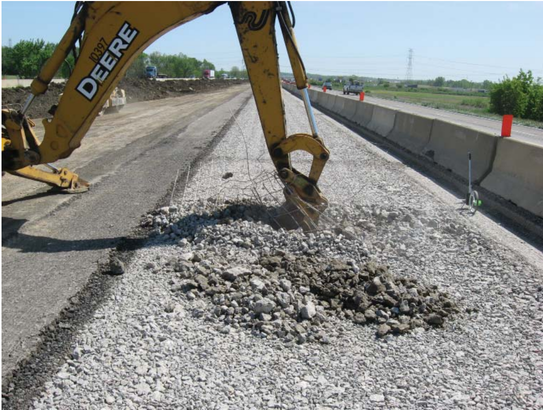
Test hole in jointed reinforced concrete pavement (JRCP).
