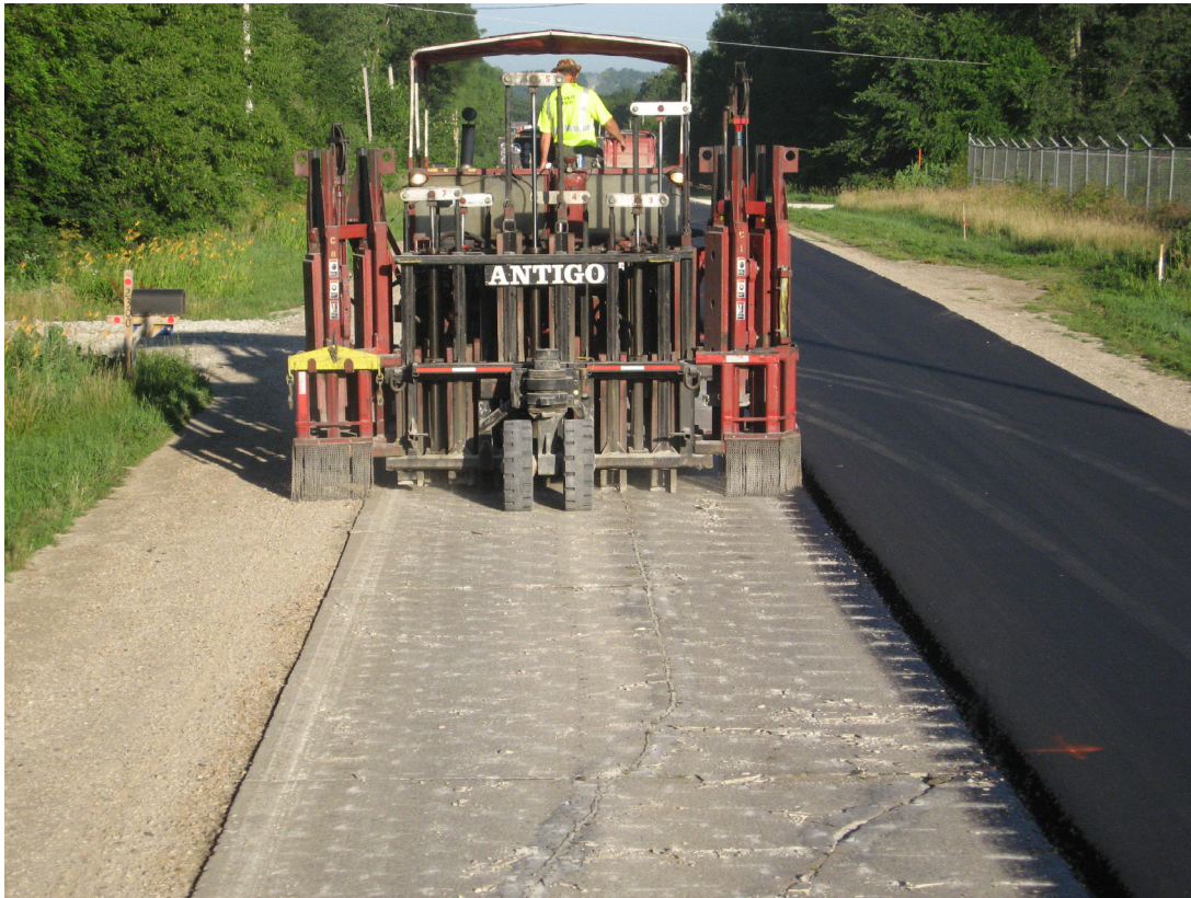
Typical modified rubblization – occasional spalling.
