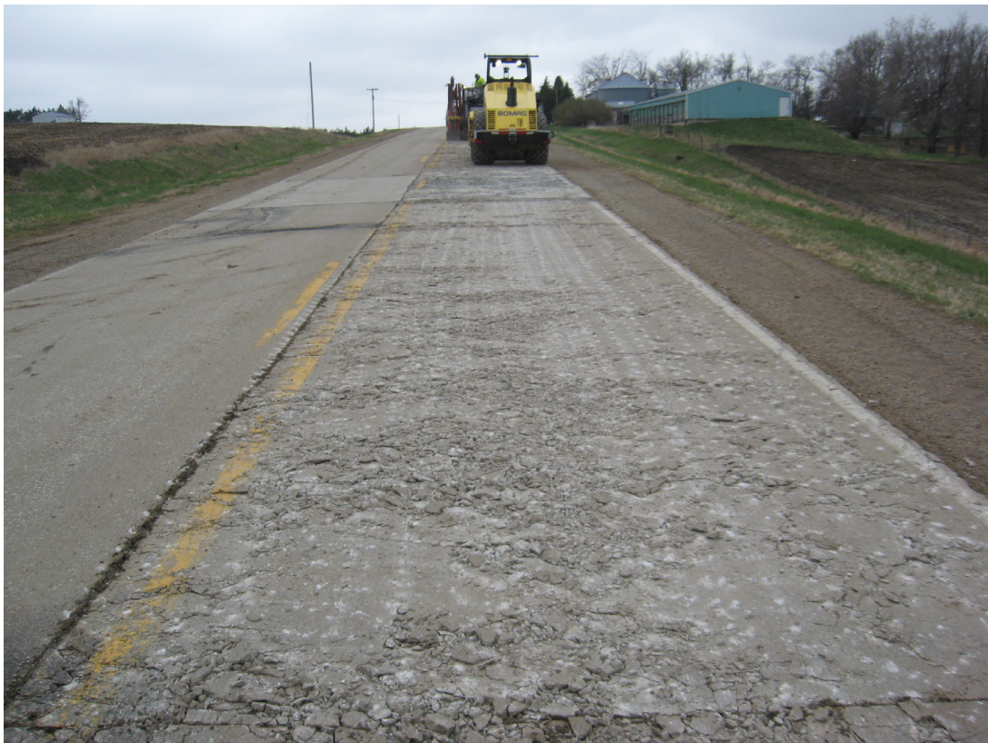
Surface after rolling with grid roller.
