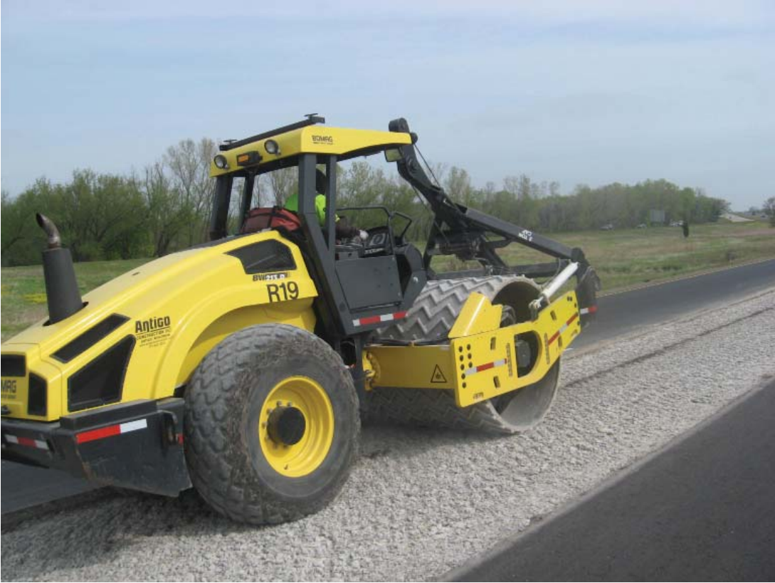
Grid roller completing breaking of surface particles.
