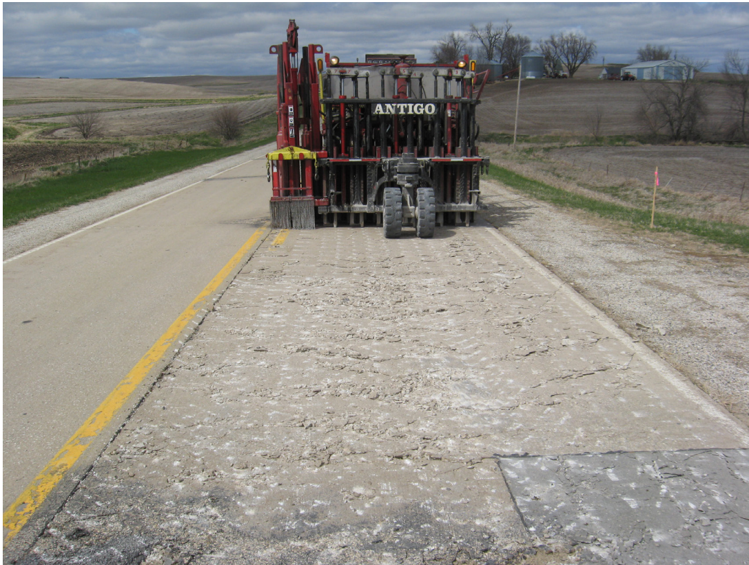
Typical modified rubblization – significant spalling.
