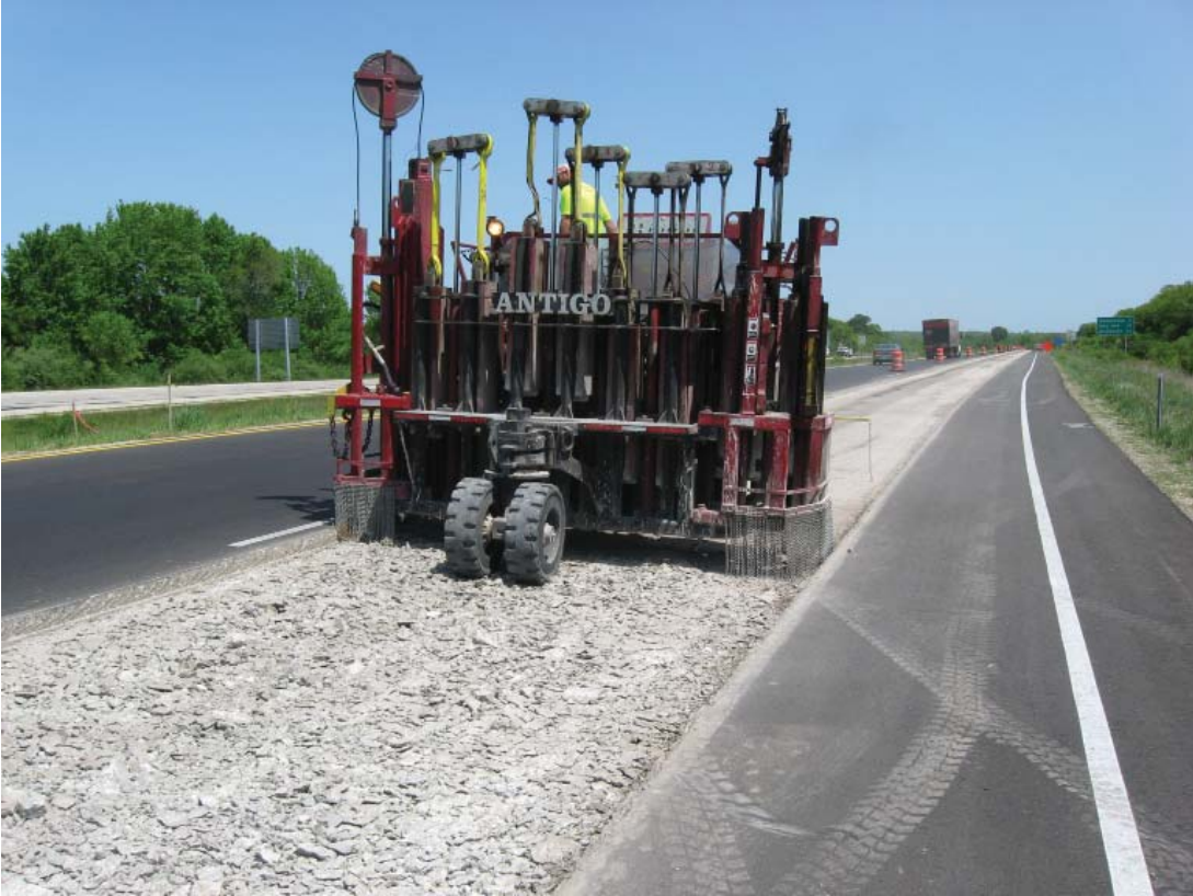
Rubblizing lane adjacent to lane previously rubblized and overlaid.
