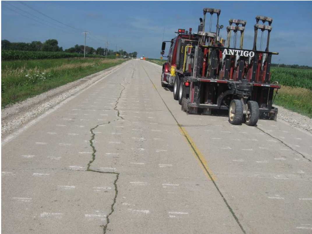
Crack and seat with MHB.
