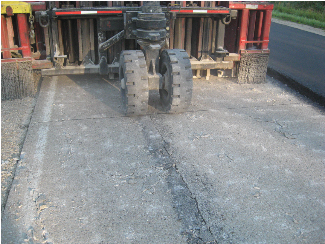
Clearly visible cracks.
