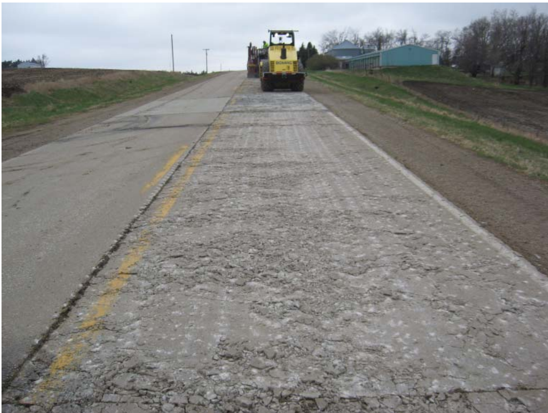
Surface after rolling with grid roller.
