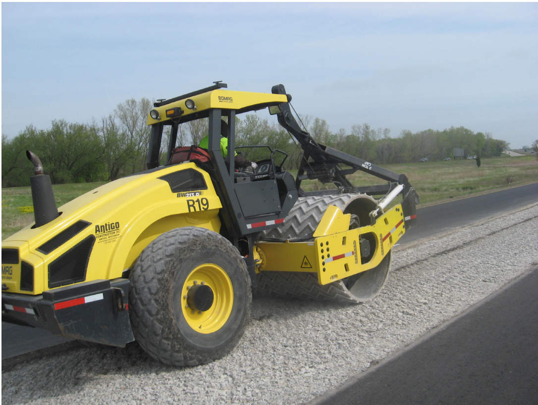
Grid roller completing breaking of surface particles.
