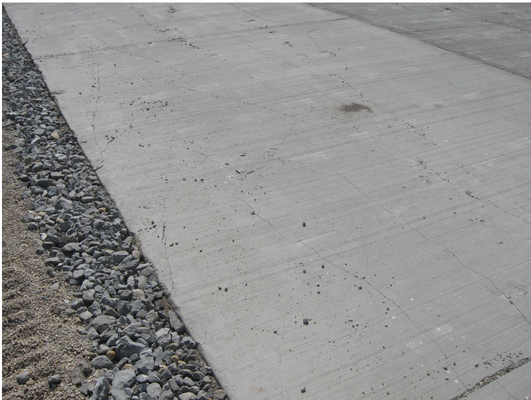
Visible hairline cracks.
