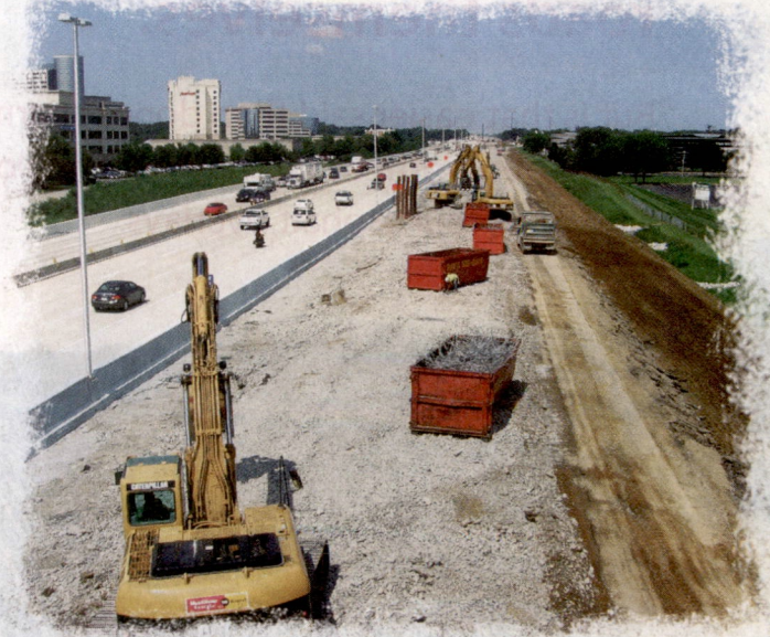
A fleet of Caterpillar excavators remove broken concrete pavement from the I-465 site.
